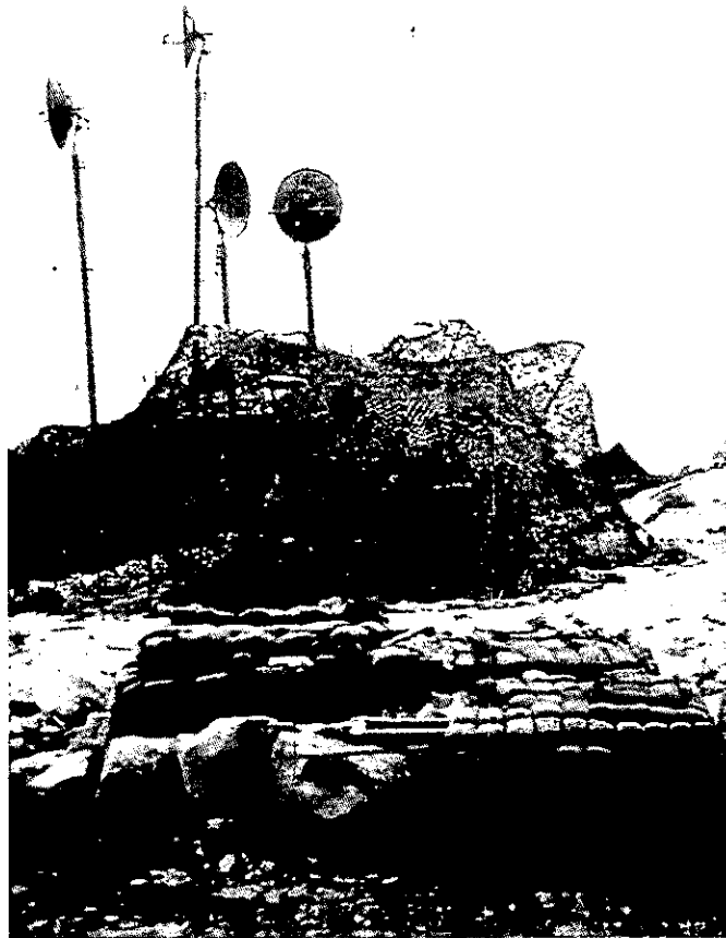
Figure K-15 Microwave Communications Relay Site Providing Communications Link Between XVIII Abn Corps and Rear Area
