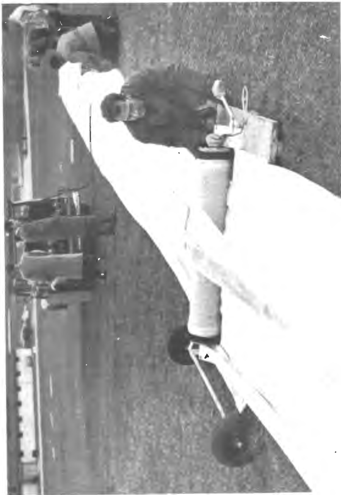
Figure 25 Launching platform with balloon fixed in place for inflation.
