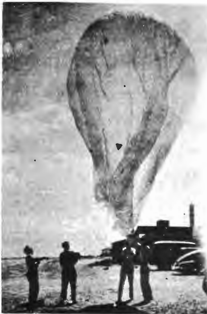
Figure 12: Neoprene balloon encased in a nylon shroud
