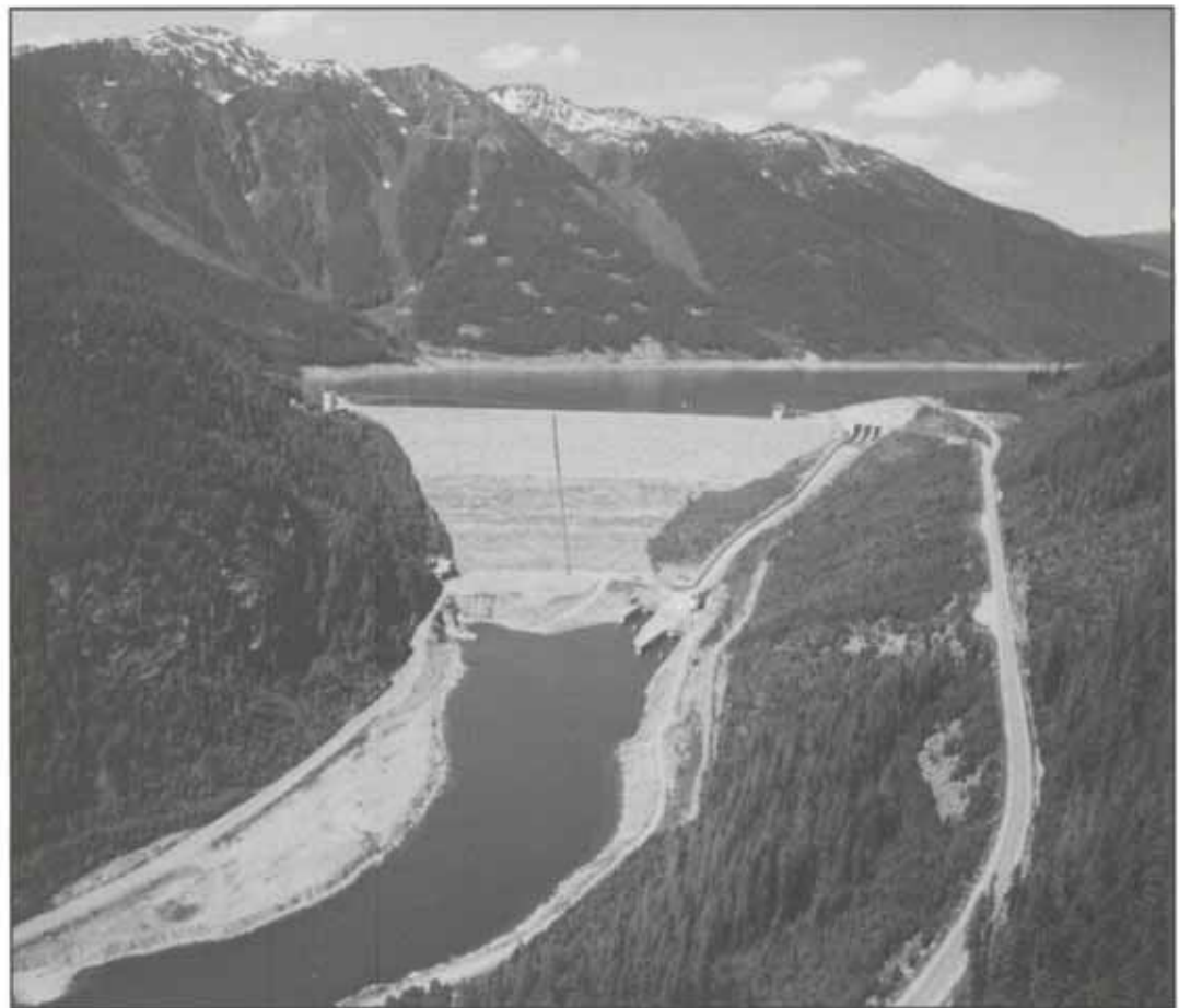
Mica Dam is one of three Canadian storage projects built as a result of the Columbia River Treaty. Canadian hydroelectric operations are among the activities not covered in the Pacific Northwest Coordination Agreement.
