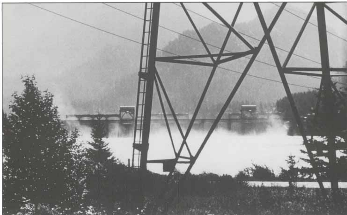
The Northwest's highly developed transmission system makes it possible to transfer power among areas with widely varying climatic conditions, electric loads and energy resources.
