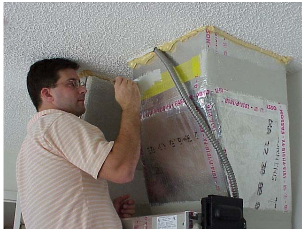
Figure 68. Supply plenum connection being sealed using foil tape, fiberglass mesh tape, and mastic.
