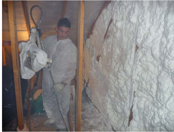
Figure 25. View of kneewall and floor cavity after being sealed with low density expansive foam.
