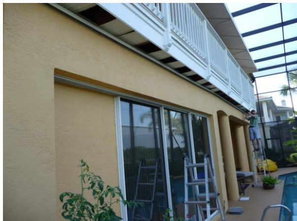
Figure 28. Soffit vent panels removed for inspection and access to seal air pathways from eave into floor cavity.
