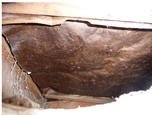
Figure 37. Insulation batts were present in most of the eave areas providing some thermal protection for the floor above. However, because the batts did not fit tightly between the joists, they allow airflow to move into the floor cavity.
