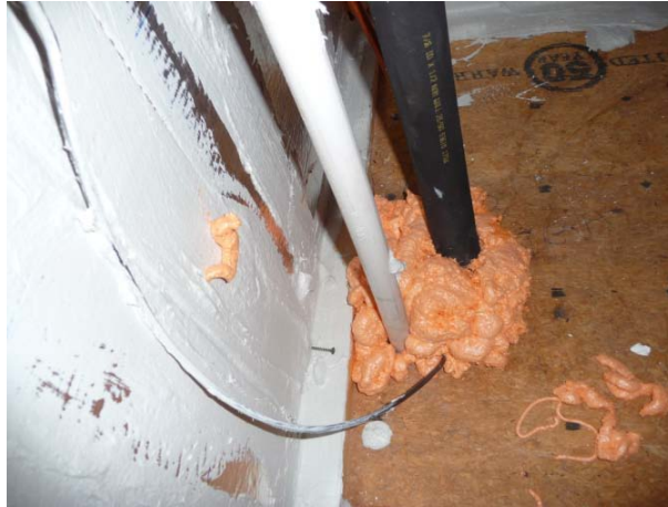
Figure 58. Penetrations in the return plenum are sealed using expansive foam.
