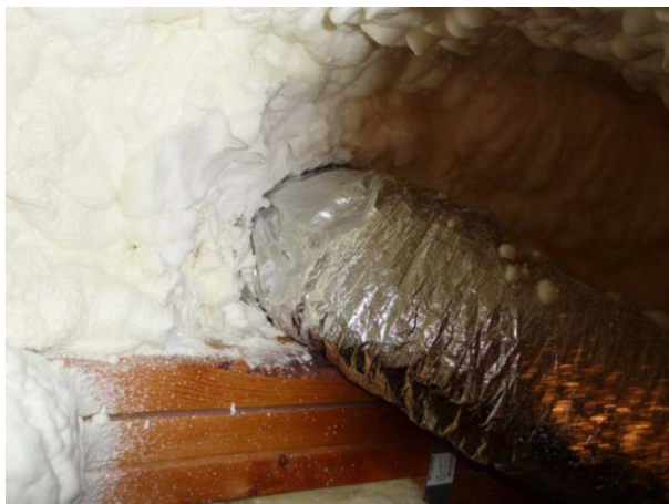
Figure 43. Supply duct from attic into floor cavity has insulation wrapped around duct before blown foam is applied.
