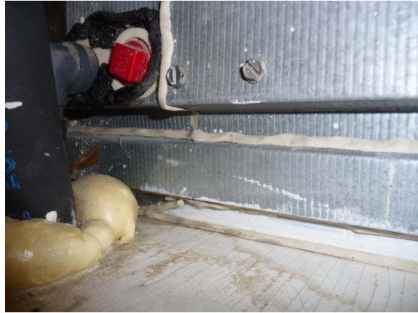
Figure 50. Black cork tape applied around condensate line penetrations and rope putty applied over seams. Expanding foam seals refrigerant line penetration into return support plenum.
