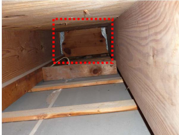
Figure 30. View from eave toward floor cavity shows pathway to floor under joist braced at back, which would be the ideal place for the air and thermal barrier in this construction.
