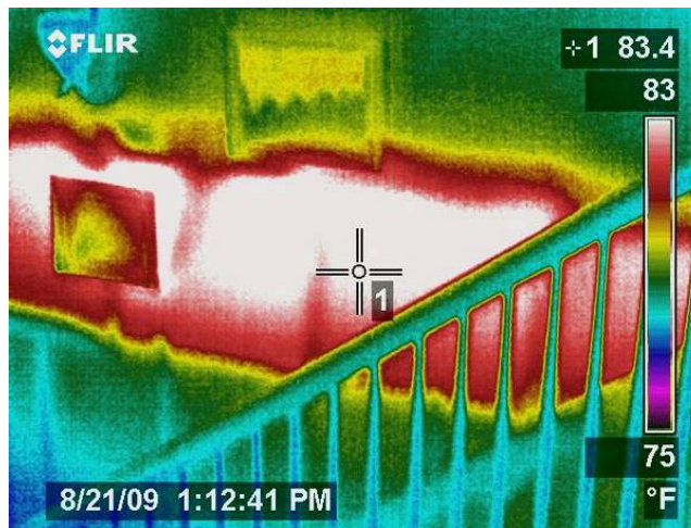
Figure 13. Infrared image of stairwell showing elevated wall temperature from hot air in an interstitial floor cavity. Note location of pictures and light fixture.
