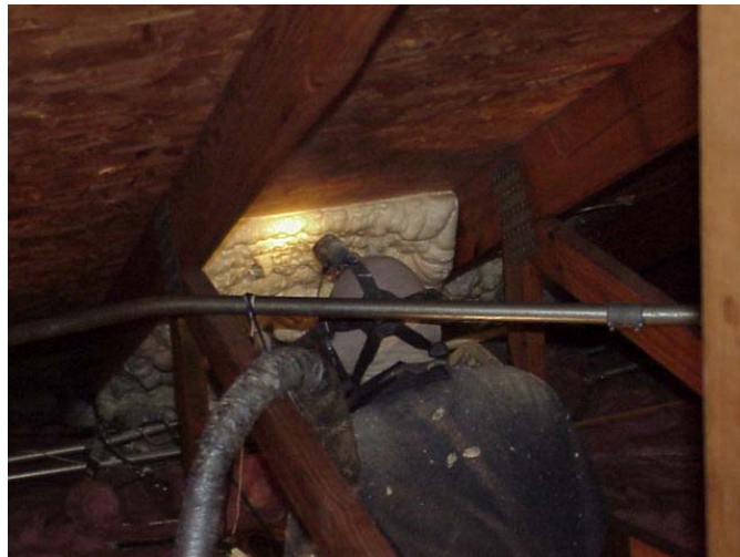
Figure 44. To encapsulate the attic space, spray foam is applied to vents and roof deck. Foam application starts low, at the top of exterior wall, sealing off the vented eave from the attic then continues to completely cover the entire roof deck.
