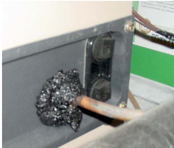
Figure 49. Black cork tape applied around refrigerant line penetration.
