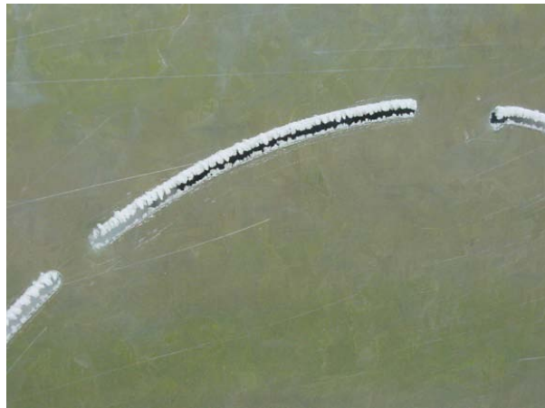
Figure 70. Sealant can be seen building on a demonstration leak.
