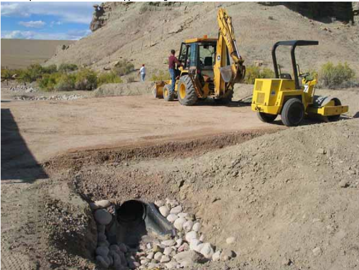
Final Inspection Photo 8 10-19-09 Upper Parking Lot
