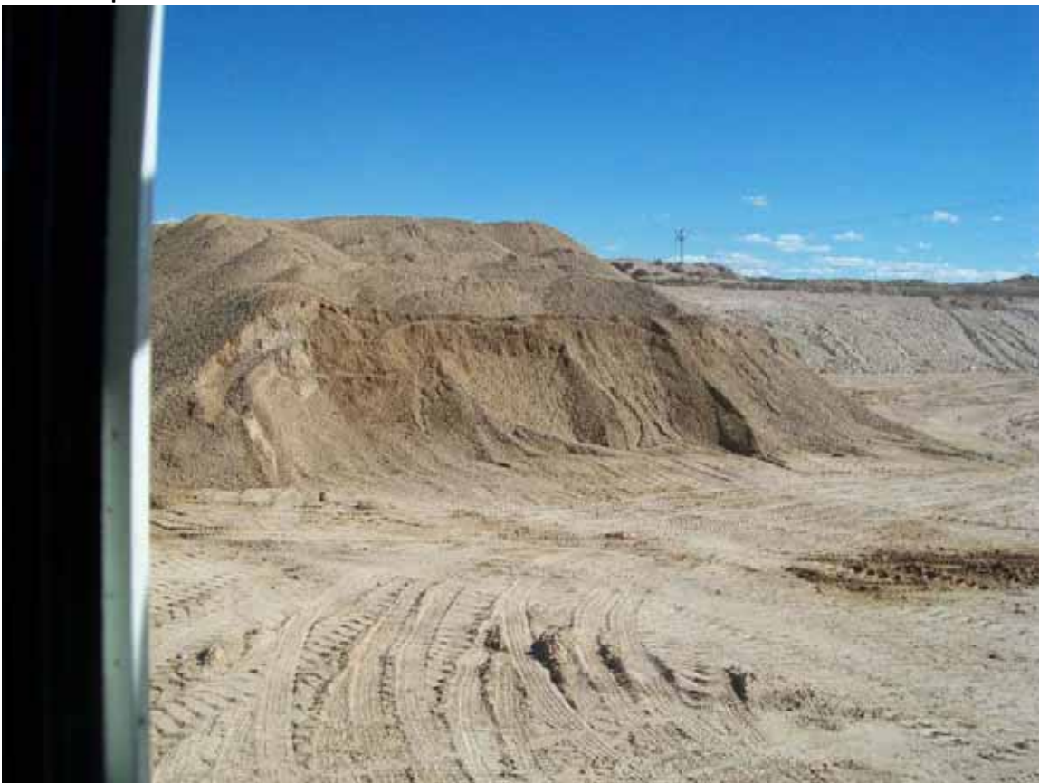
Interim Inspection Photo 6 10-15-09
