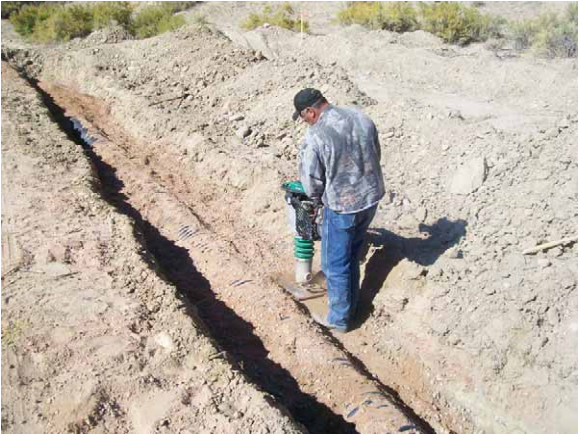
Interim Inspection Photo 3 10-15-09
