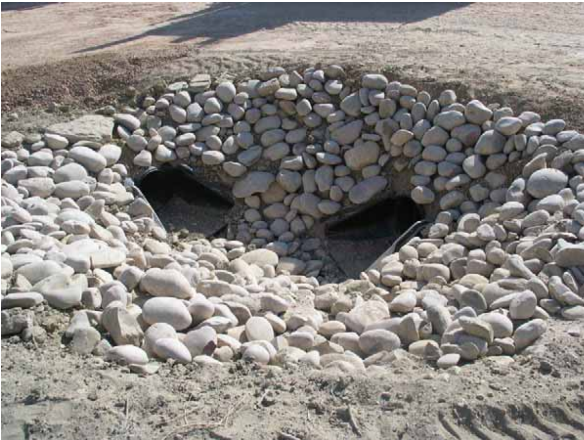
Final Inspection Photo 7 10-19-09 Upper Parking Lot
