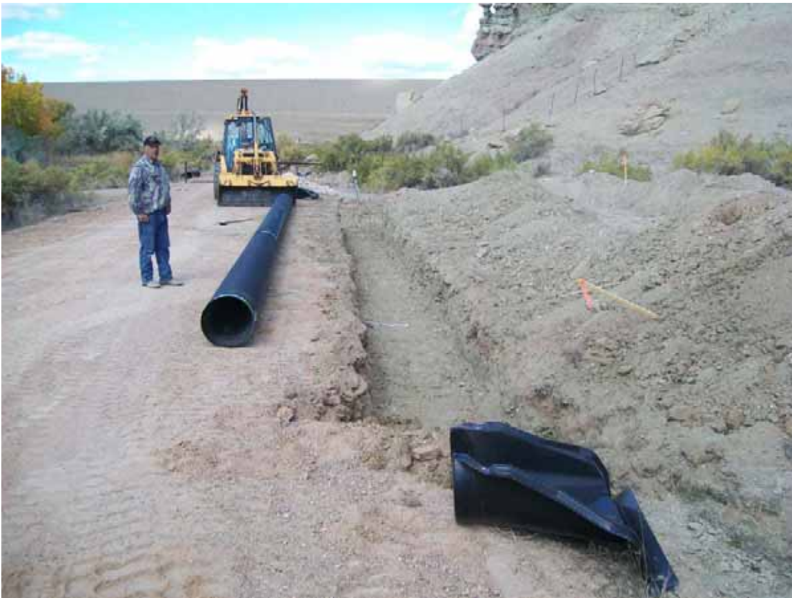
Interim Inspection Photo 1 10-15-09
