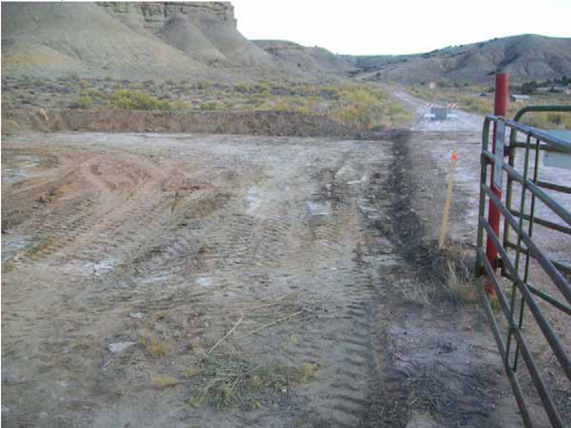
Interim Inspection Photo 4 10-15-09
