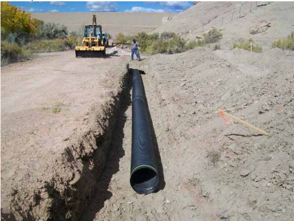
Interim Inspection Photo 2 10-15-09
