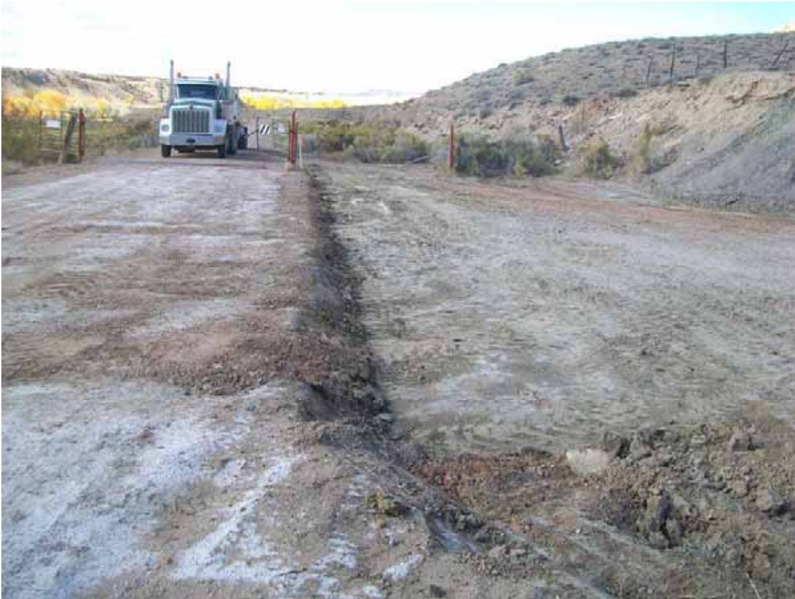
Interim Inspection Photo 5 10-15-09
