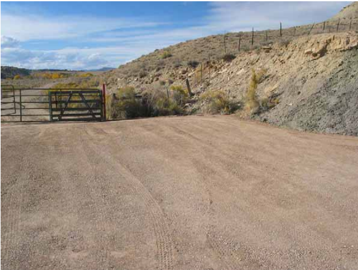
Final Inspection Photo 9 10-19-09 Lower Parking Lot
