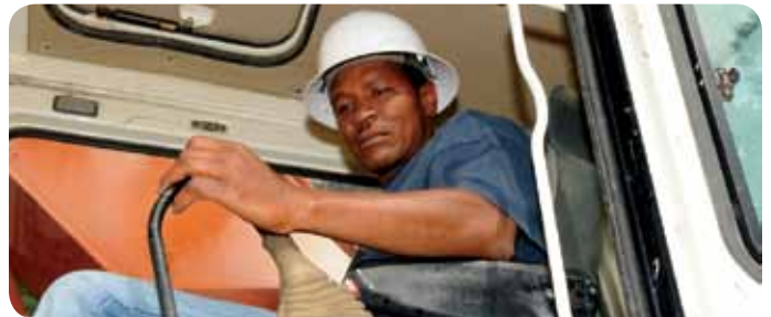
Mike Dale operates construction equipment for the new wastewater treatment plant.
