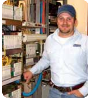
The VTCI project will use equipment similar to what is shown above.
