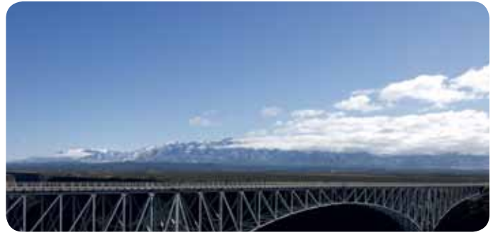
Residents around the Rio Grande Gorge Bridge, located in Taos County, will be offered broadband service.
