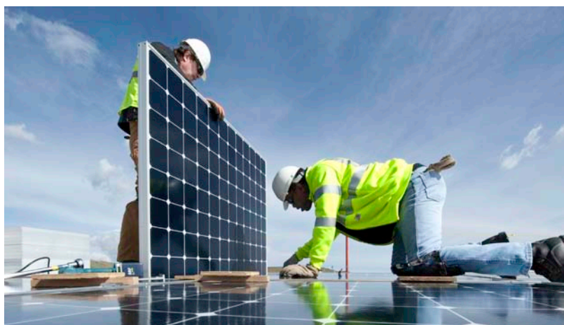
Photo by Dennis Schroeder, NREL/PIX 21499
