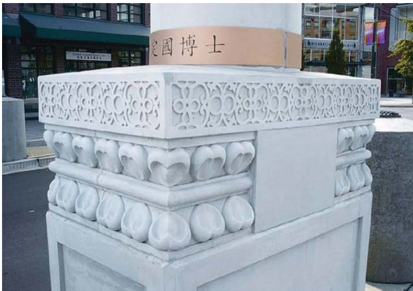
Figure 1: SCC easily fills precast forms
