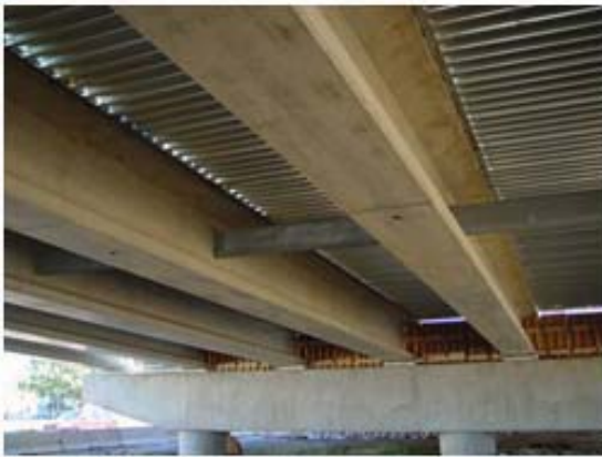
Figure 4: SCC girders support the PRB [13]
