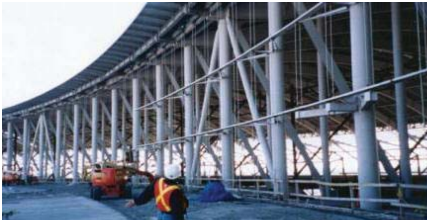
Figure 2: SCC can be pumped into hollow steel tubular columns [12]
