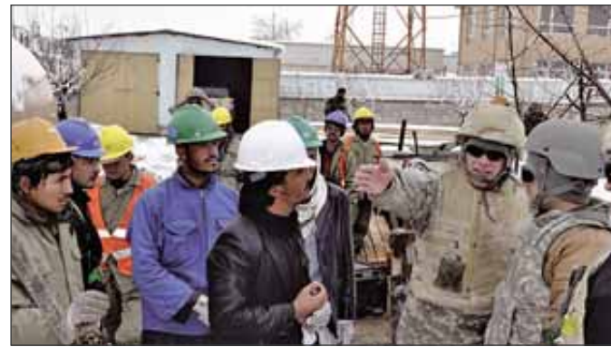
Philip Kielhurn, project engineer and contracting officers' representative with the U.S. Army Corps of Engineers Afghanistan Engineering District-North, speaks with a local site supervisor and workers at the Afghan National Army Recruiting Center in Pul-e Alam, Feb. 13.
