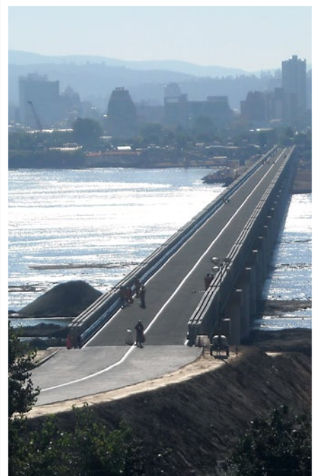
Acrow Corporation modular bridge in Chile.
