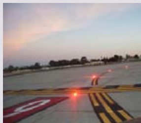
RWSLs are used to hold takeoffs, as well as to signal when aircraft may or may not enter a runway.
