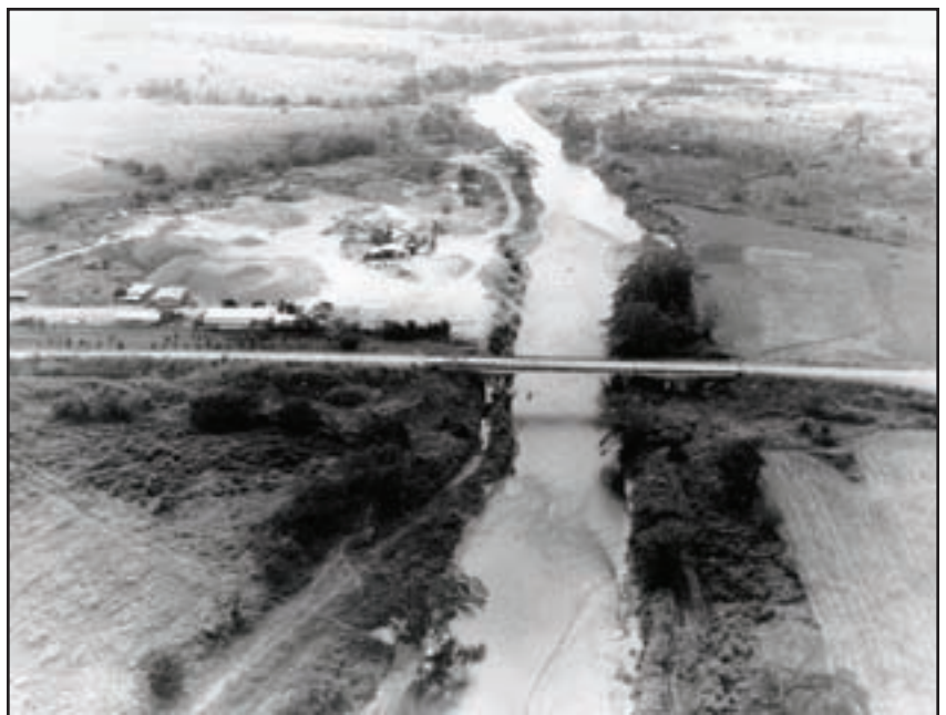
Pacora River Bridge.
