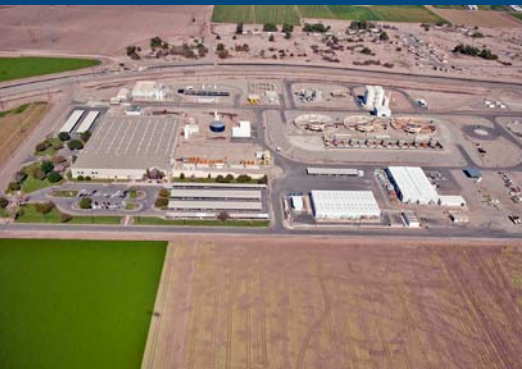
Aerial view of the Yuma Desalting Plant complex.
