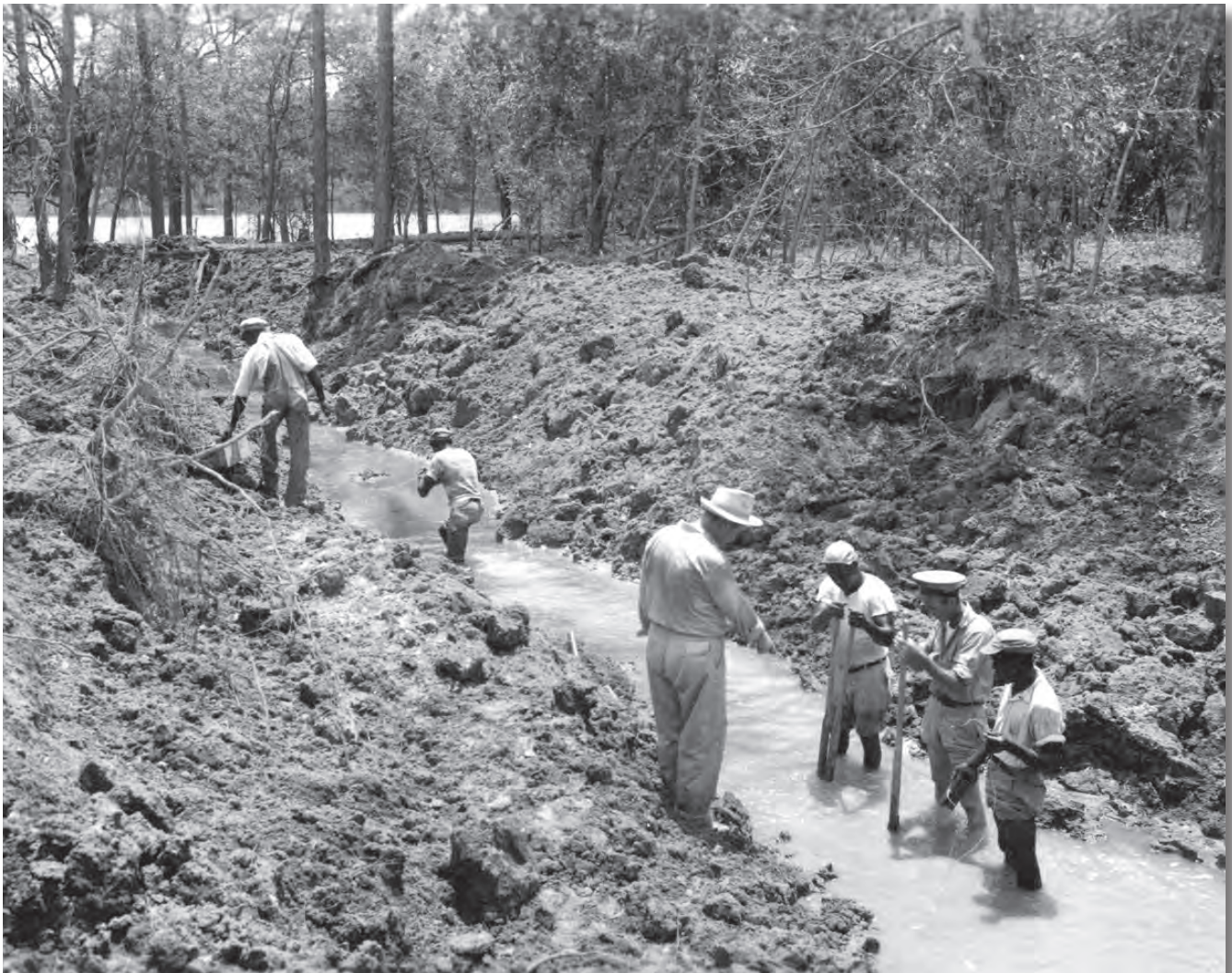
The floods in Florida in 1948 were fought using drainage canals to divert water from towns, roads, and farmland. Workers placed explosive charges to expand Malone Canal near Marianna, Florida.
