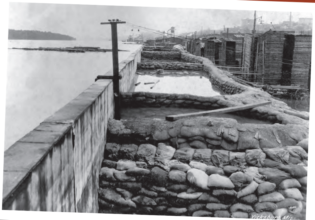
Right: Sandbag cells reinforced a locally-built floodwall at Vicksburg, Mississippi, on 3 May 1927.
