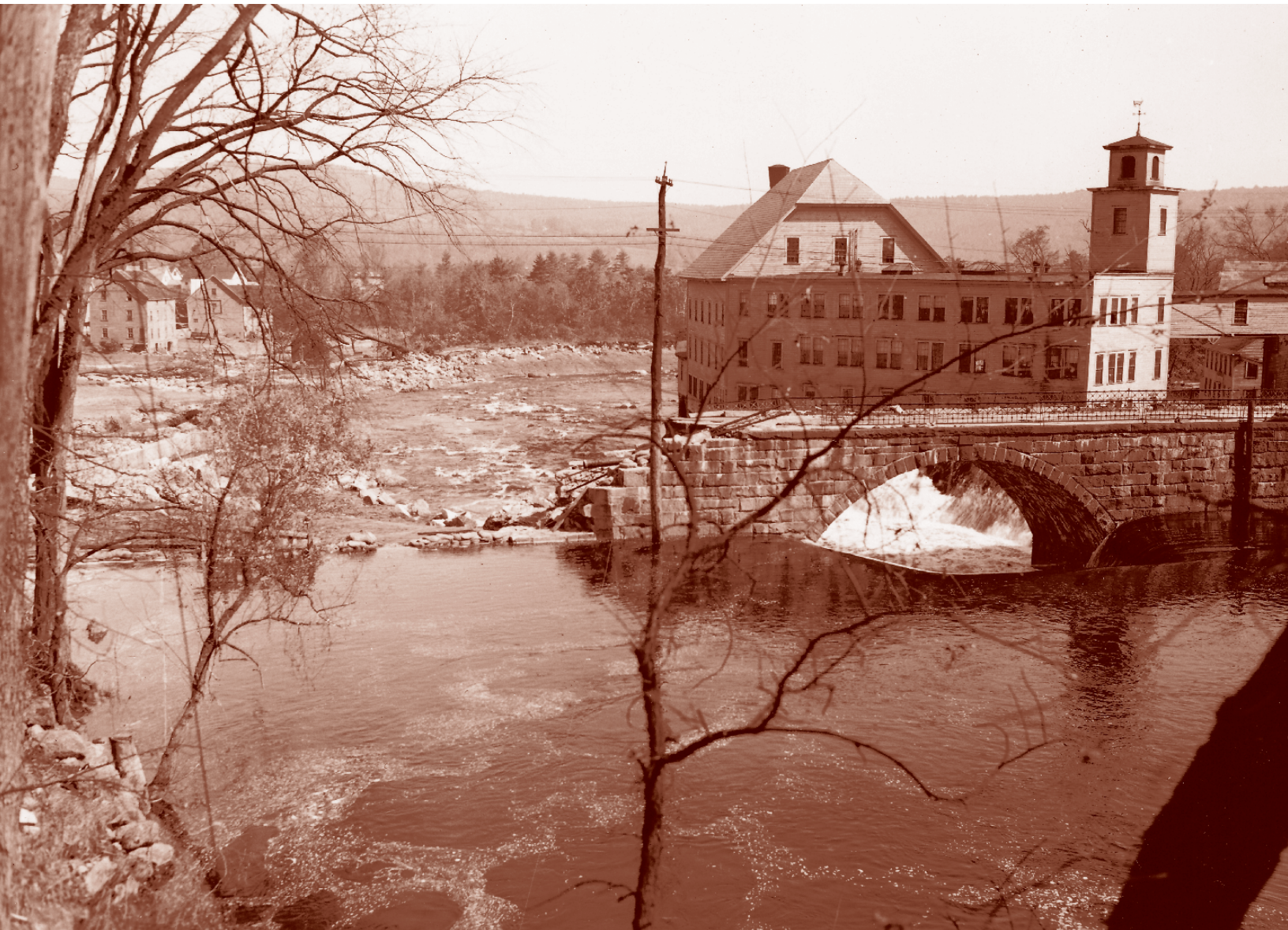
A stone bridge in Hillsboro, New Hampshire, was swept away by flooding and wind from the September 1938 New England hurricane.
