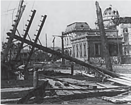
The hurricane that hit Galveston in 1900 also destroyed Corps facilities and killed Corps employees. Library of Congress, LC-USZ62-78468
