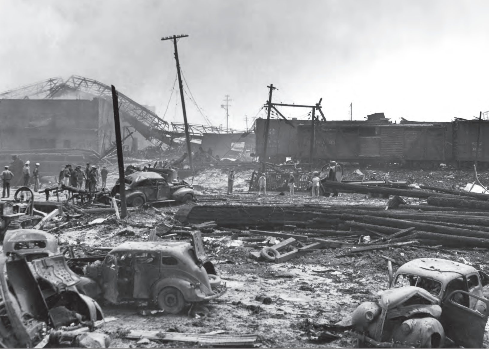
After the explosions and fires, the Texas City railroad yard was filled with destroyed vehicles and buildings.
