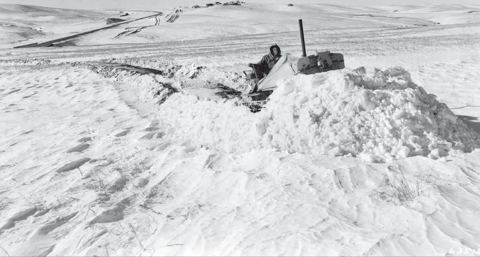
An Army bulldozer cleared snow from a road near Pierre, South Dakota. The Army coordinated more than one thousand bulldozers and heavy tractors used to help reach stranded towns, ranches, and livestock.
