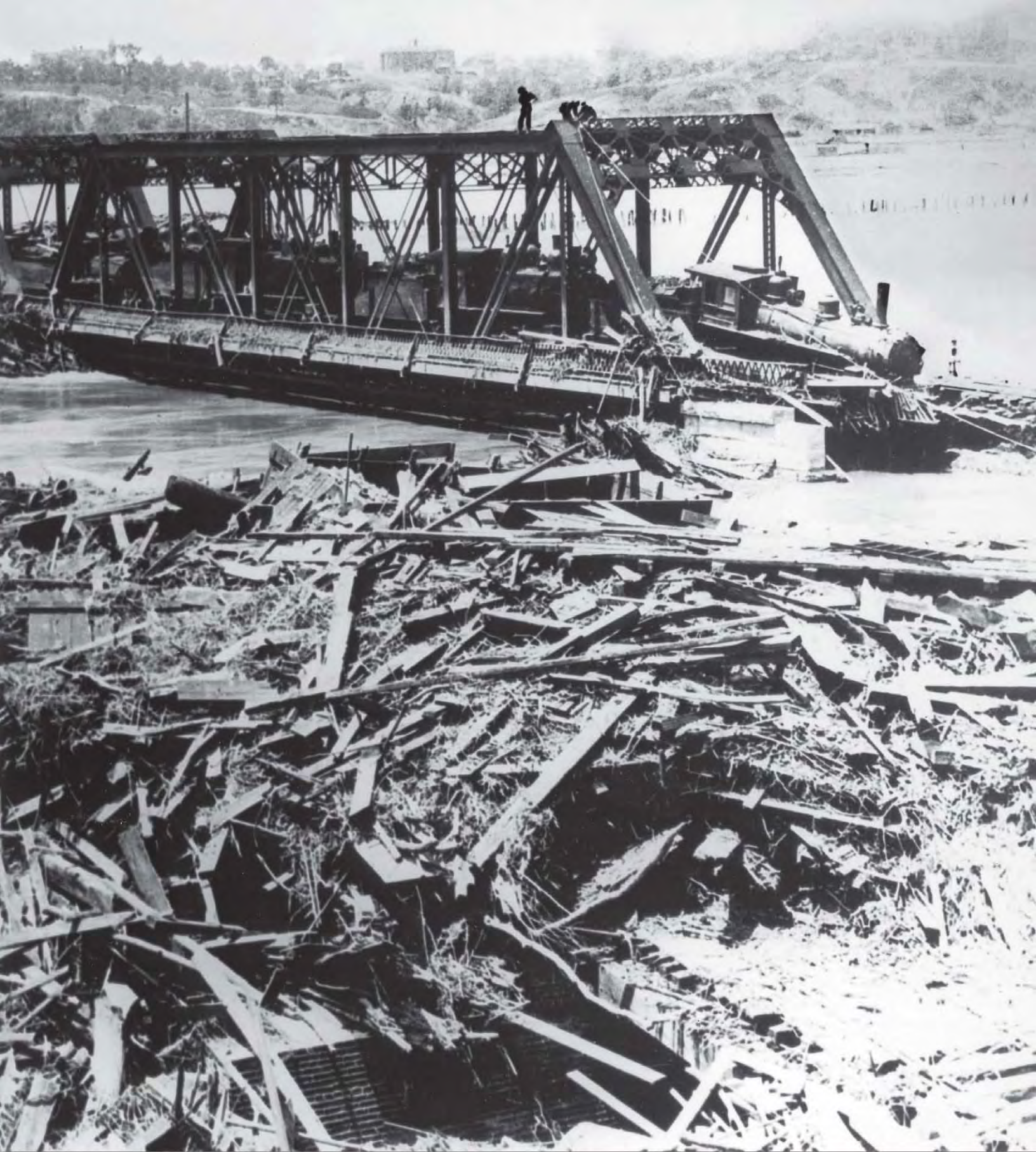
During the 1903 flood at Kansas City, locomotives parked on the Missouri Pacific Railroad bridge helped prevent the flood and debris from taking out the bridge.
