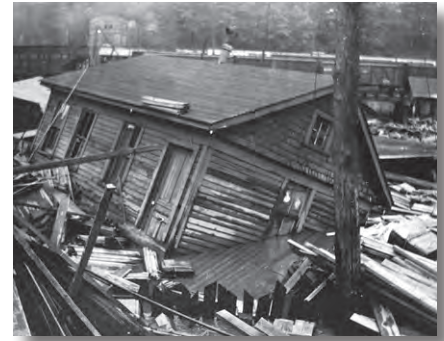
Torrential rains in 1916 caused damage to Asheville, North Carolina.
