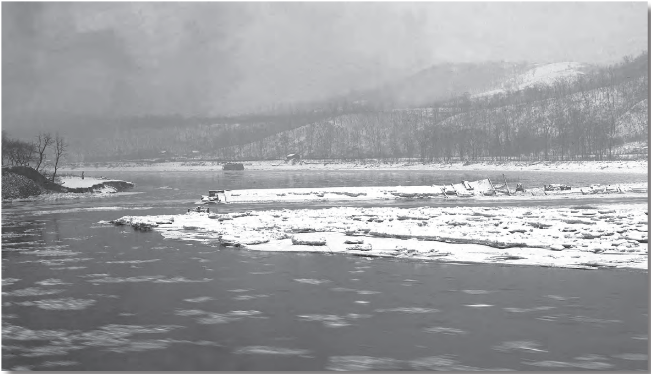
In 1907 the Corps of Engineers broke open Dam 3 on the Allegheny River to prevent bank erosion and property damage. The remnants of the dam are in the foreground.
