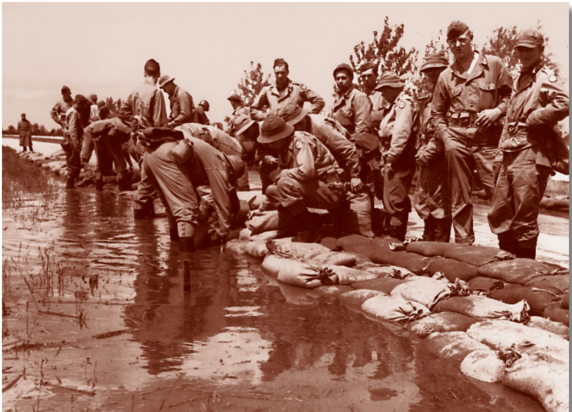
Army troops placed sandbags along the Illinois River near Beardstown, Illinois, during the 1943 flooding.
