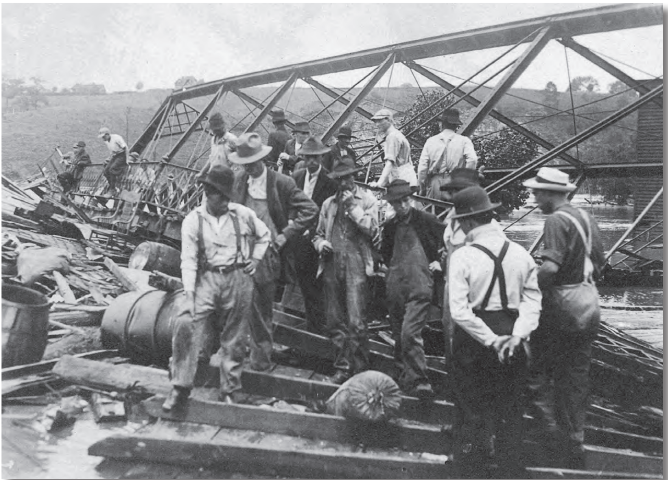
Residents milled around on a damaged bridge in Asheville, North Carolina, 1916.
