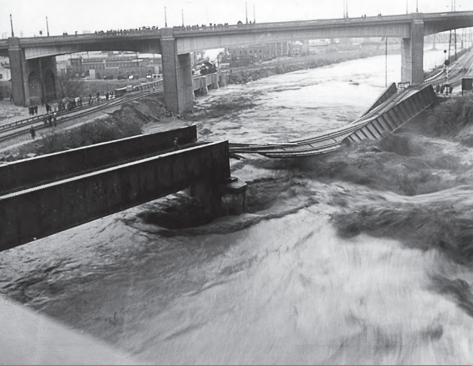
The May 1938 flood of the Los Angeles River destroyed this railroad bridge in downtown Los Angeles.
