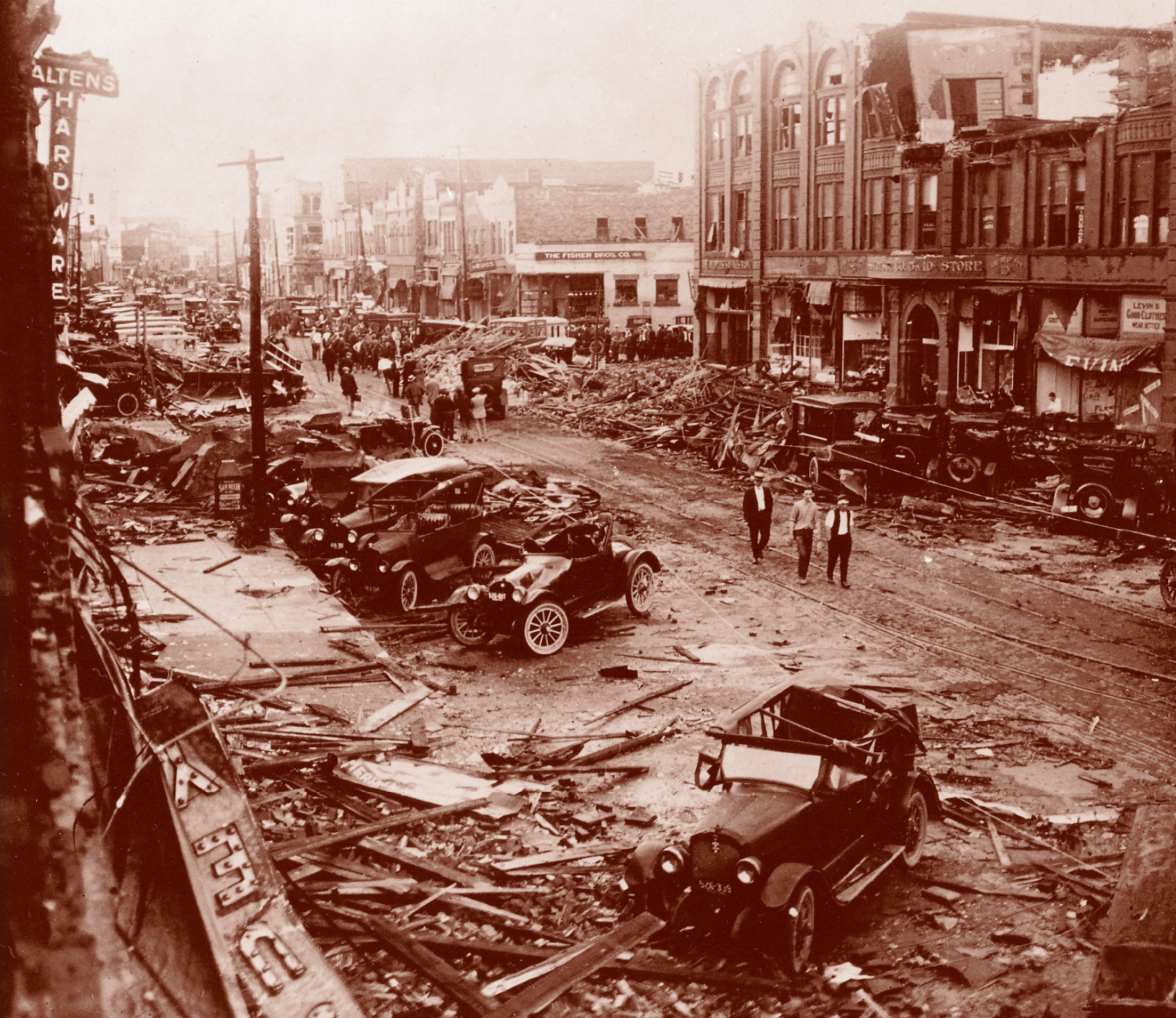
A tornado severely damaged Lorain, Ohio, on 28 June 1924.
