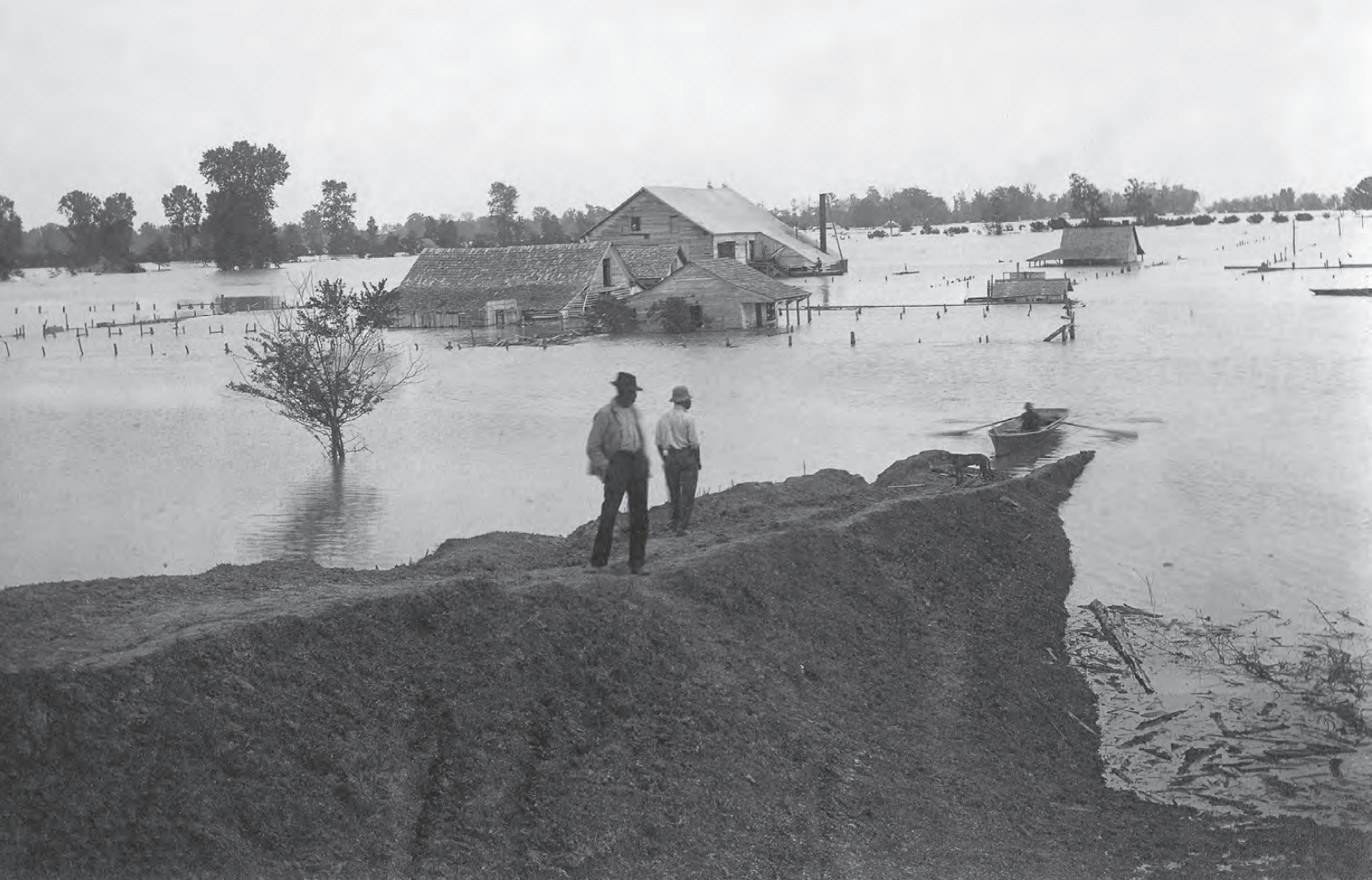
W. H. Brown's gin house, two miles above the Skipwith crevasse at Addie, Mississippi, succumbed to floodwaters in 1913.
