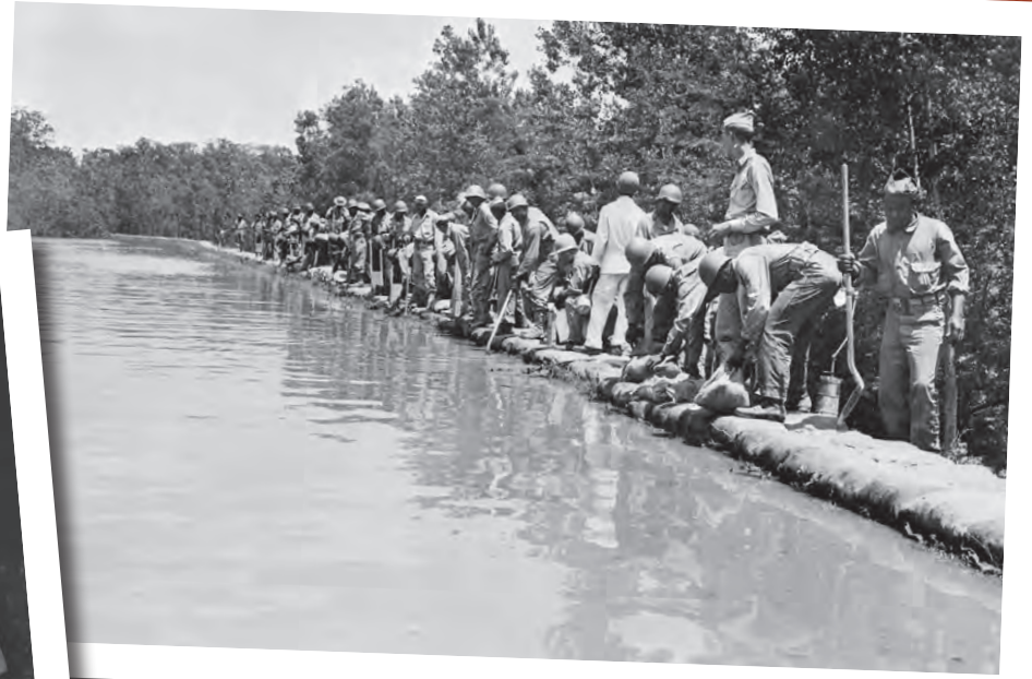
Above: A levee at Sand Mills, Arkansas, was reinforced by members of the 354th Engineer Regiment, May 1943.
