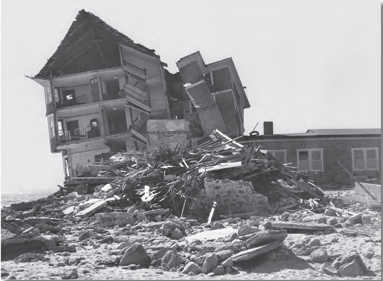
The hurricane that struck New England in September 1938 left part of the Pleasant View Hotel on Misquamicut Beach, Rhode Island, standing precariously in the rubble.
