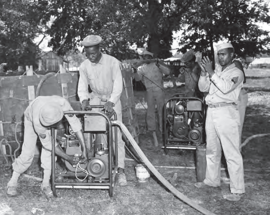
During the May 1943 floods of the Missouri and Mississippi river systems, soldiers were mobilized to shore up the levee on the White River at Peach Orchard Bluff, Arkansas. Water purification equipment operated by the 364th Engineer General Service Regiment provided drinking water to the troops.
