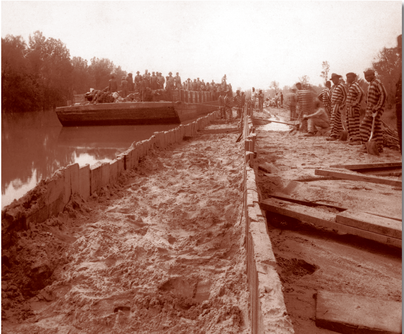
Convicts constructed a mudbox atop a levee near Fulton to hold out the Mississippi River flood in 1927.
