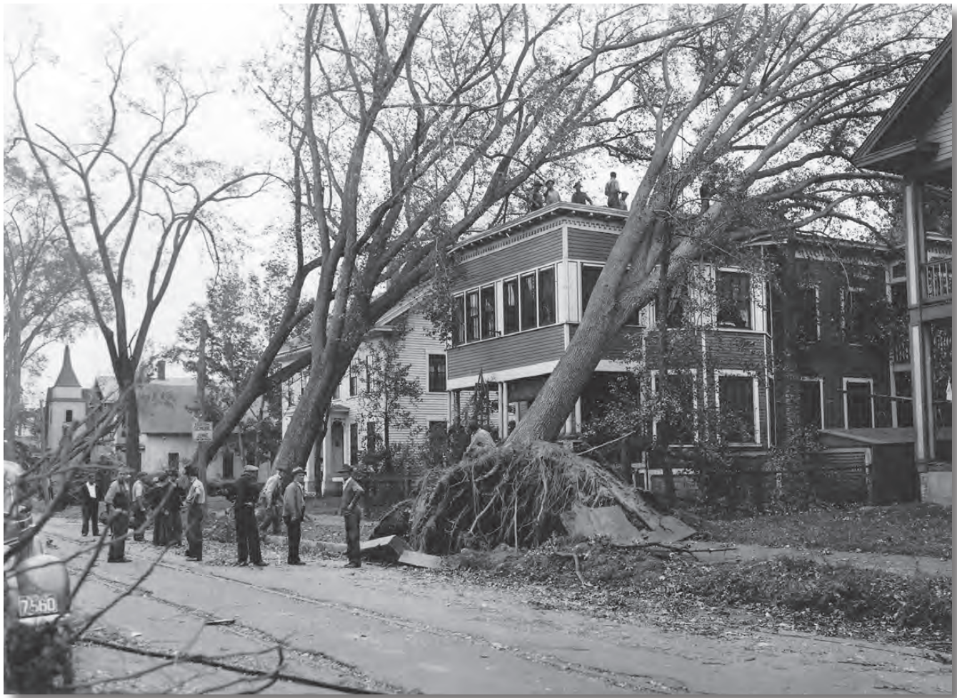
Trees on Manchester Street in Manchester, New Hampshire, were uprooted and toppled by the 1938 hurricane, damaging a number of buildings along the street.
