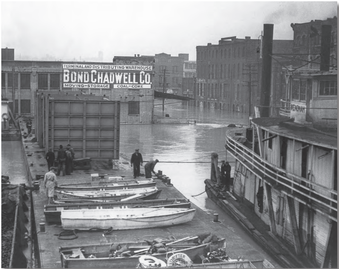
Engineers loaded rescue craft in flooded Nashville, Tennessee, 1937.
