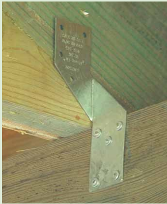
Figure 4-3. This is the popular H2.5 hurricane clip installed during new construction of houses. Five nails are hammered into the lower beam (or top plate) and five more need to be used for the roof (truss-rafter) connection. A hurricane clip is required for each truss-rafter. Upon completion of this structure, the hurricane clip will be hidden from view. This particular clip costs 30 cents. For less than one dollar in material cost, stronger ones can be installed for both new and retrofit applications.
