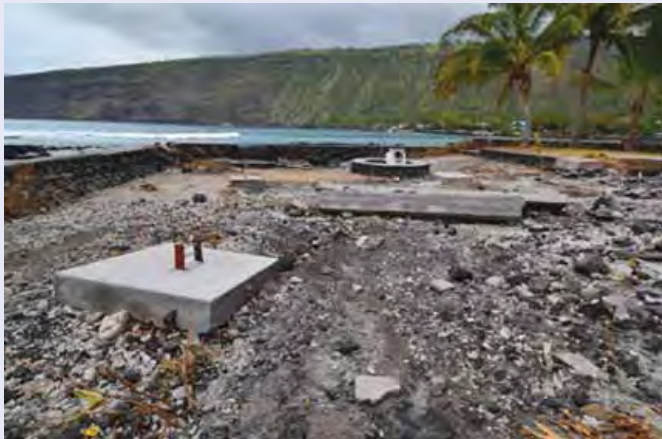
Figure 2-2. The tsunami generated from the March 11, 2011 earthquake off Japan damaged many residences in Kealakekua Bay on the island of Hawai'i. The house on this empty lot was swept into the bay.
