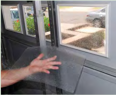
Figure 4-22. Laminated film comes in various thicknesses and strengths. Here the film is applied to an existing window before it is fastened to the frame with silicone structural sealant.
