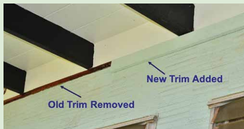
Figure 4-11. The old trim has been pulled. The new trim is 1 inch x 4 inch exterior wood, treated for termites, painted with primer and two coats of paint that color match the wall. Color matching can be done by taking a small sample to your local hardware store.
