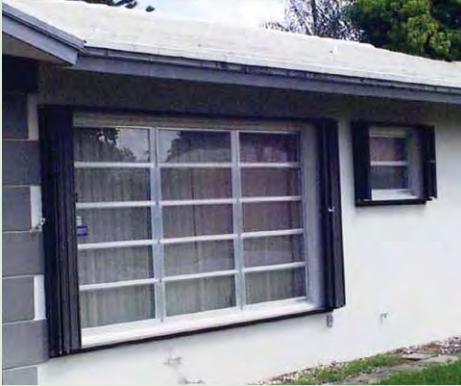
Figure 4-18. For deployment during a storm, the panels unfold accordion-style and extend toward the center of the window along pre-installed tracks. Photo courtesy of the Department of Emergency Management, City and County of Honolulu.
