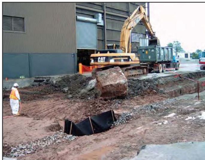
Linde Site Excavation
