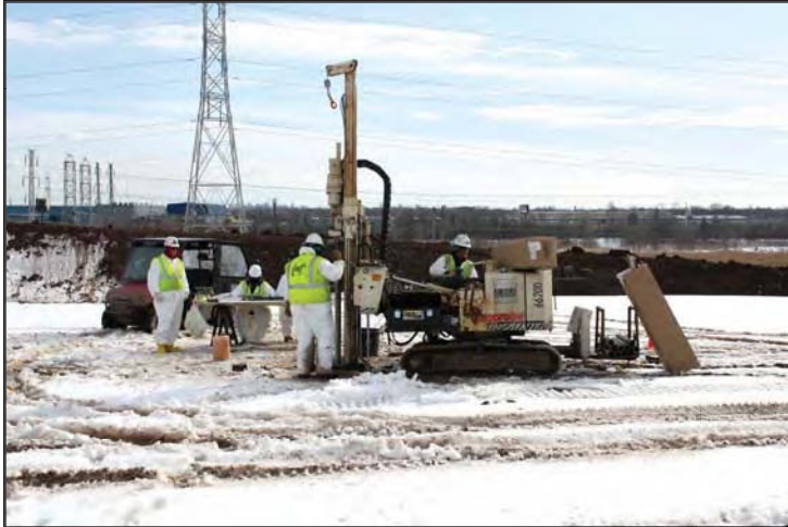
Tonawanda Landfill Soil Sampling
