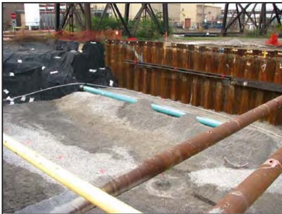
St. Louis Downtown Sewer Replacement
