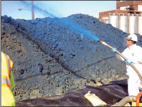
Painesville Site dust control agent application
