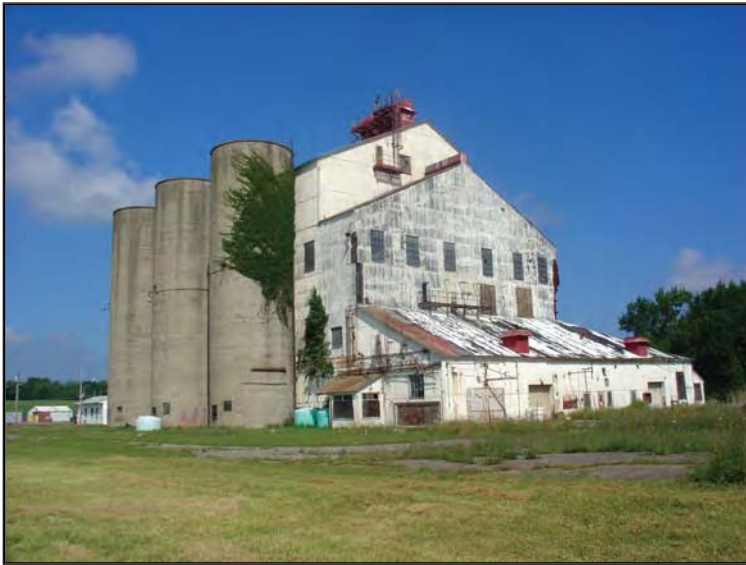
Niagara Falls Storage Site Building 401
