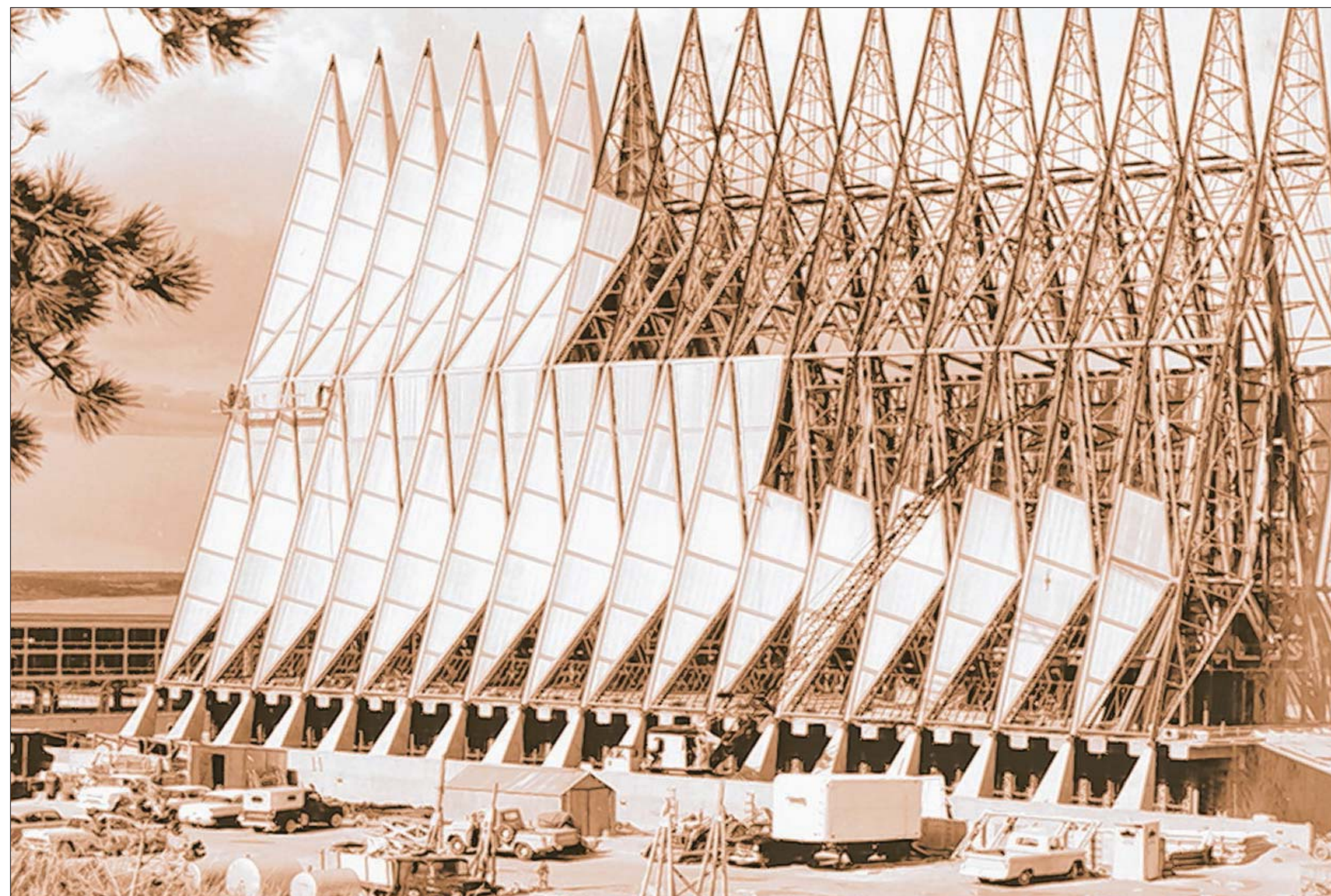
The Air Force Academy's iconic chapel was completed in 1963 and dedicated on Sept. 22, 1963. The chapel cost $3.5 million in 1959 dollars and is now the most visited man-made attraction in Colorado.
