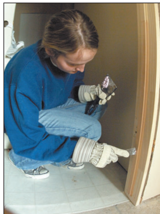
Left: Cadet 3rd Class Rehling Hitt of CS-22 spackles an interior doorway. Right: Cadet 3rd Class Trevor Boyd of CS-23 sands a light socket, to prepare a room for painting in the home of future homeowner Rachel Vasquez of Montrose.
