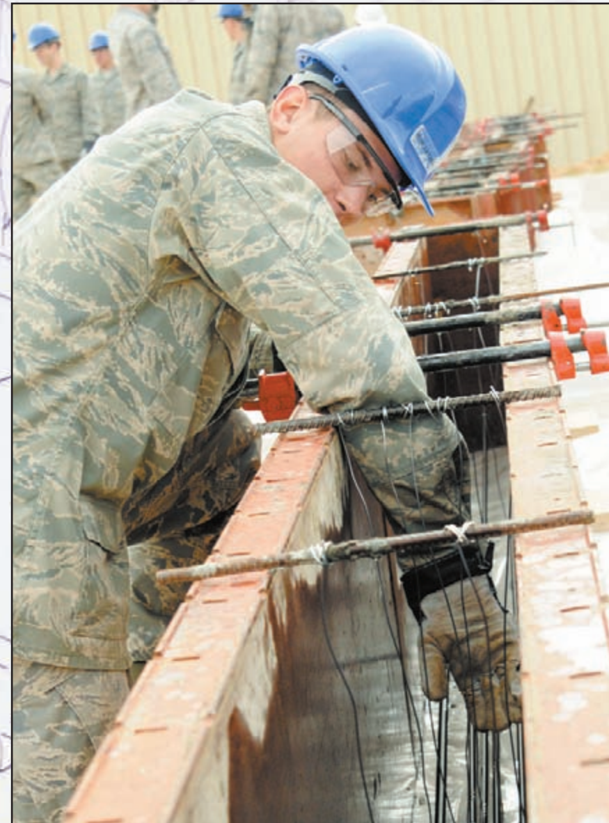
Right: Cadet 2nd Class Casey Habluetzel adjusts the rebar during concrete beam pouring.
