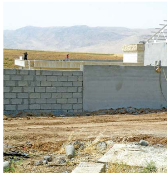
Partially completed security fence surrounding the abattoir.
