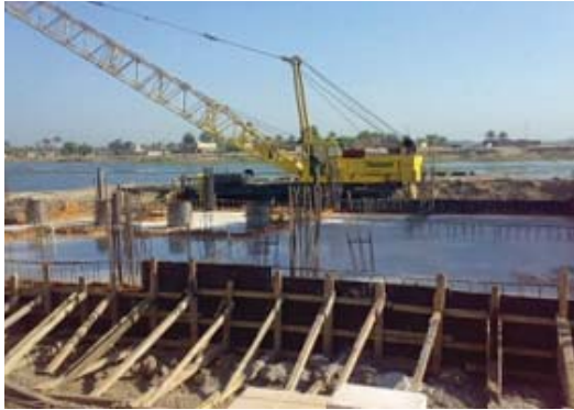
Construction continues on the Meshkab Water Supply Project. (GRD photo)
