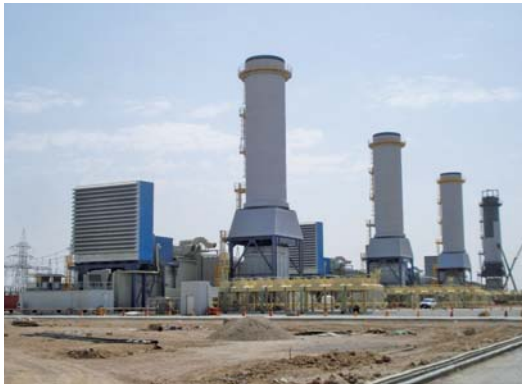
The Erbil Gas power plant, privately built and operated, had an average output this quarter of 368 MW, which is 75% of its nameplate capacity. (KRG Ministry of Electricity photo)
