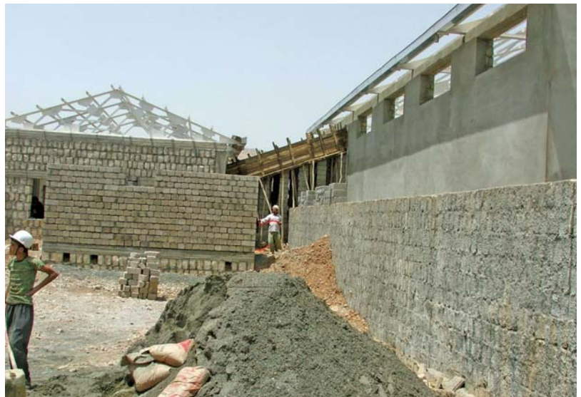
Ongoing construction at the abattoir.
