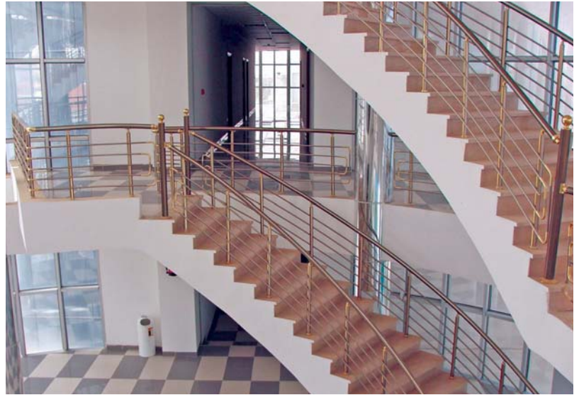
Central rotunda primary stairwell.
