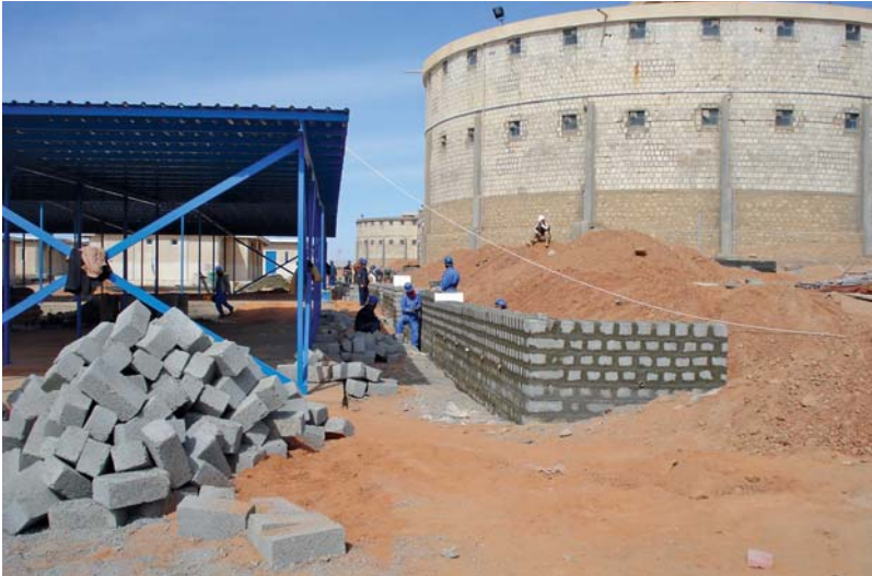
Ongoing construction at Chamchamal.
