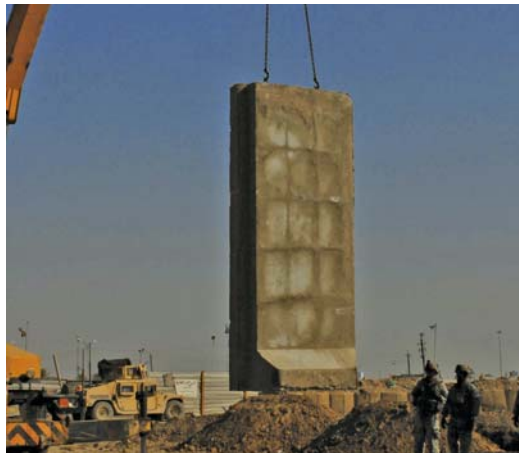
A concrete blast barrier, known as a "t-wall," being emplaced in Baghdad. (MNF-I photo)
