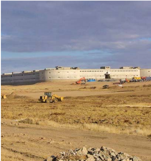
Ongoing construction at Chamchamal site.
