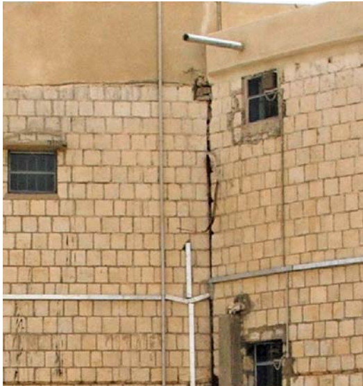
Pre-existing external expansion joints.
