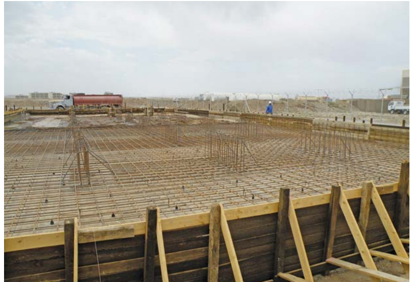
Raft foundation for benzene storage at Al Kasik.
