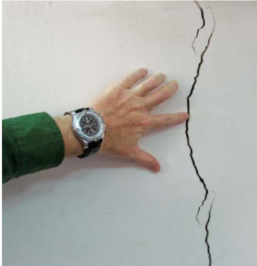
Settling crack.
