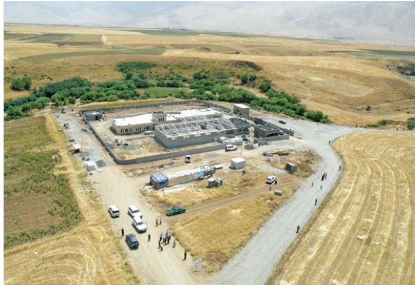
Aerial overview of the abattoir project.
