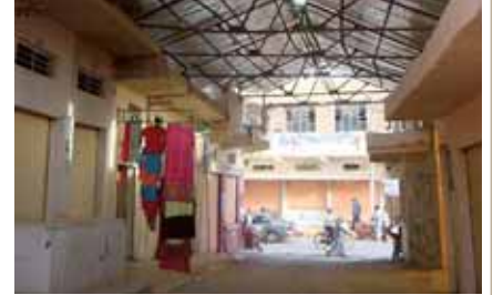
Diyala suq refurbished with U.S. assistance.
