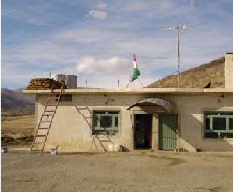
Front exterior of border post
