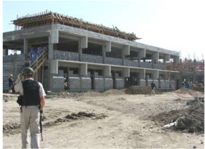
One of the prison inmate housing units under construction
