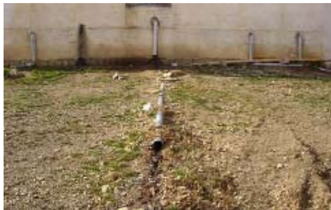
Sewer outfall behind border post at MNSTC-I border post
