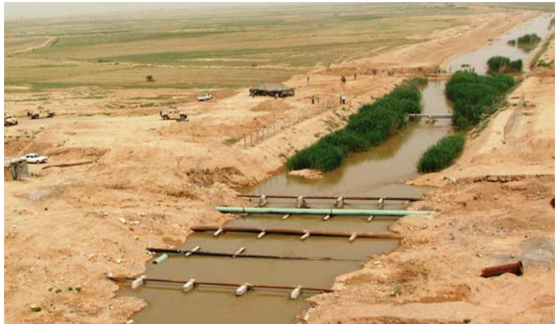
Aerial view of Zegeton Canal Crossing (with old pipelines visible)
