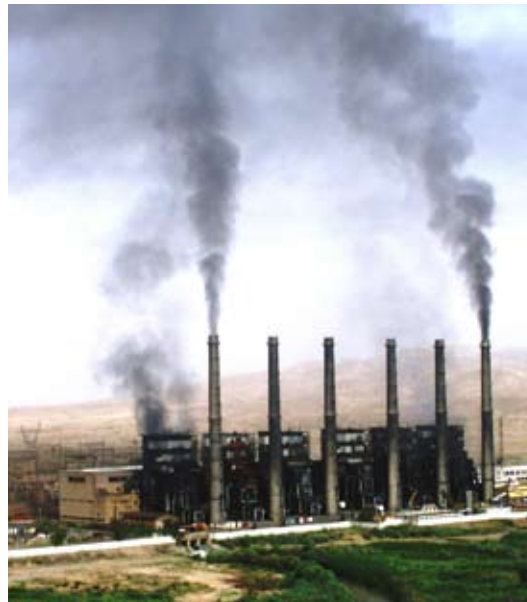
Baiji Power Plant
