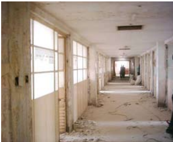
View of interior partitions before refurbishment (photo courtesy of USACE)
