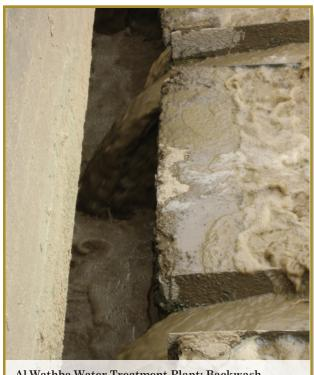
Al Wathba Water Treatment Plant: Backwash effluent, a portion of which enters the clear well tanks and then the Baghdad drinking water system.
