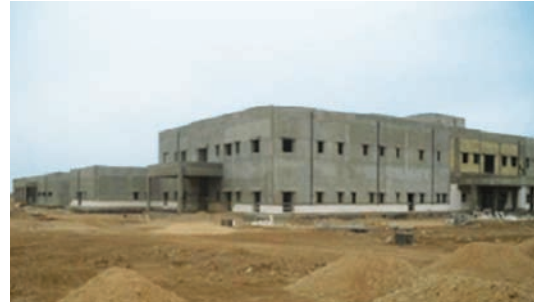
The Missan Surgical Hospital as it looked on December 12, 2010. (USACE photo)
