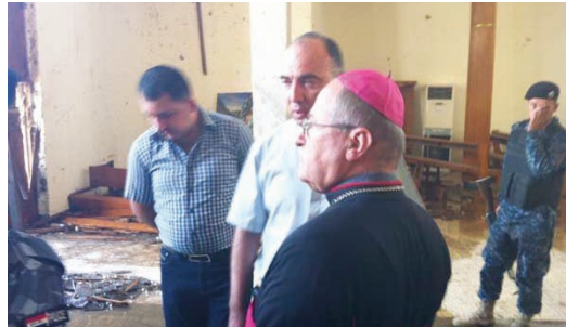
GOI and church officials survey the damage after the October 31, 2010, attack on Our Lady of Salvation Church in Baghdad. (Ankawa photo)
