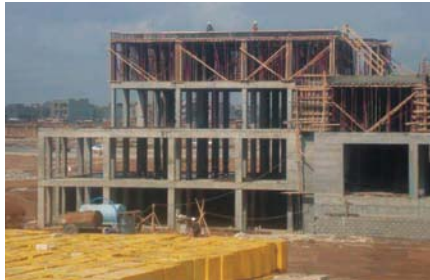
Construction of Emergency Hospital in Erbil City. (OPA photo)
