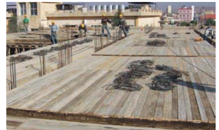
Construction of Emergency Hospital in Zakho City. (OPA photo)
