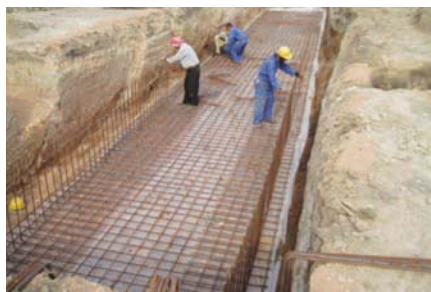
Laying groundwork for the Al-Khidhir slaughterhouse. (OPA photo)
