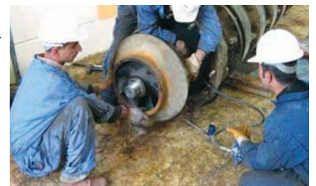
Disassembling a vertical turbine pump in Sulaymaniyah. (OPA photo)
