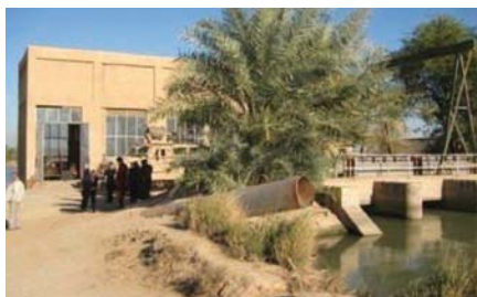
As Shuahmiyah Pump Station. (OPA photo)
