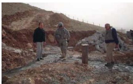
Construction of artesian water wells. (OPA photo)
