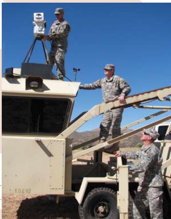
(L-R): Electronics technicians Staff Sgt. Wayne Rogers, Spc. Larry Hill and Sgt. 1 st Class Fred Beauchemin install a "4-Eyes" remote camera system atop a Sky Tower near Sasabe, Ariz. The "4-Eyes" system has telescopic and infrared capabilities which allow Soldiers from distant locations to monitor the illegal aliens as they cross the U.S. border from Mexico.
