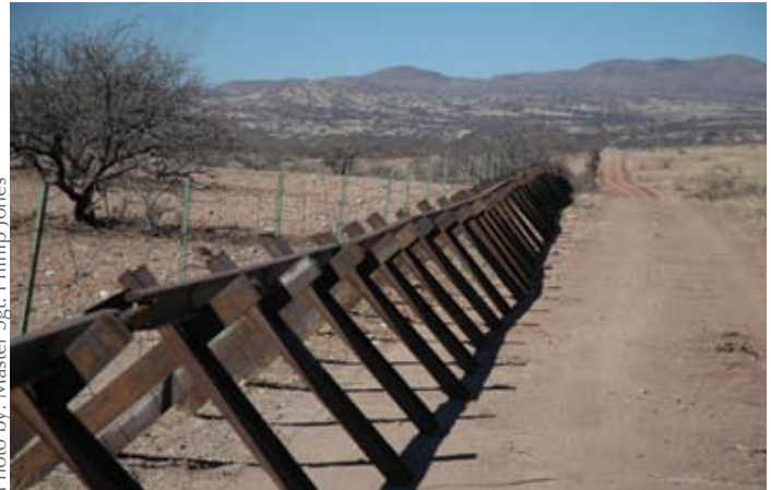
This vehicle barrier fence built by the 122 nd Engineers is an effective way to prevent Mexican drug cartels from driving their shipments into the U.S. along remote, desert areas of the border.
