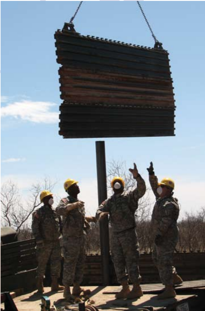
(L-R) Spc. John White of Lexington, Spc. James Penderhill of Rock Hill, Spc. Antwan Hemphill of Rock Hill and Spc. Tim Worthy of Rock Hill guide the landing mat into place.
