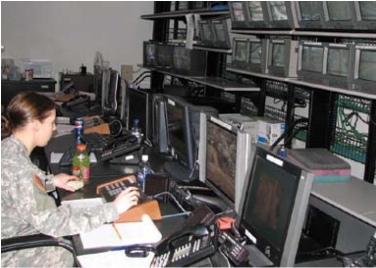
National Guardsmen help staff Border Patrol communications centers like this one in Nogales, Ariz. Utilizing sophisticated communications, sensor and camera surveillance systems to supplement the S.C. National Guard's entry identification team sites and aviation assets, the U.S. Border Patrol is able to put more agents on the border to apprehend illegals and cut off the flow of illegal narcotics into the U.S.
