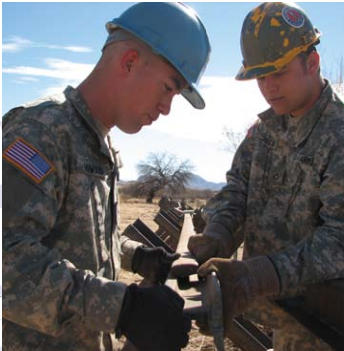
(L-R): Spc. Joe Howard of Aiken and Pfc. Brandon Corley of Newberry place a "Key" between two links of a vehicle barrier they are helping build along the Mexico border in Sasabe, Ariz. Each 25-feet of vehicle barrier weighs approximately 1,500 lbs.
