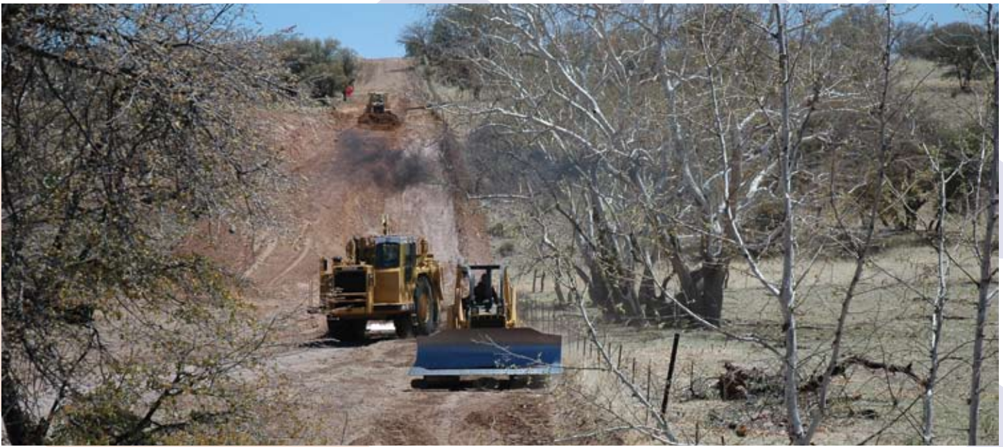
(L-R): Nearly a mile above sea level, the 178 th Engineer Battalion begins moving a hill to create a flat road in a treacherous wash along the border fence separating the U.S. and Mexico.
