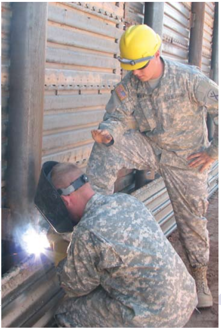
(L-R): Spc. Chris McQueen of Ft. Mill and Pfc. James Miller of Rock Hill weld a landing mat into place.
