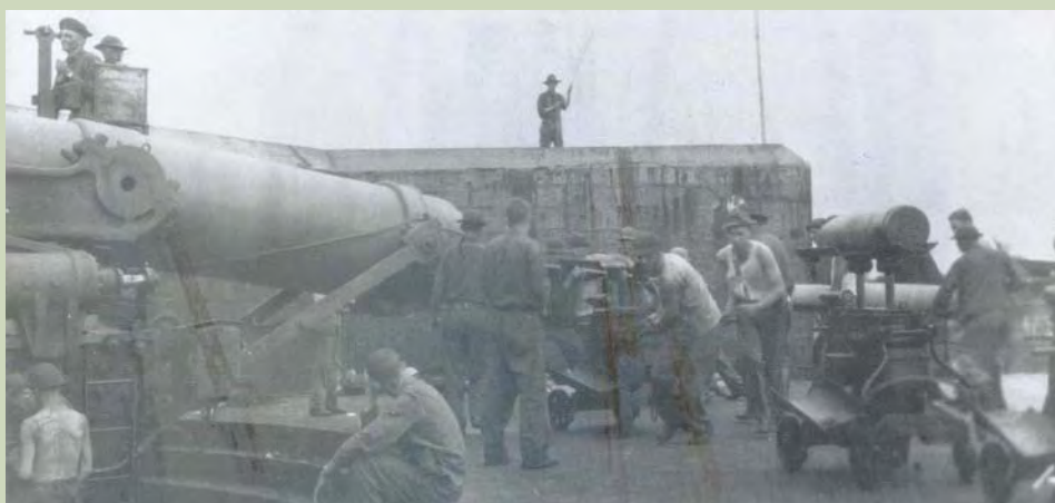
S.C. National Guard Coastal Artillery Soldiers practice firing one of four 10-inch rifles mounted on disappearing carriages. When fired, the rifles recoiled behind Battery Jasper's walls at Ft. Moultrie.
