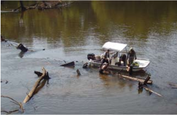
Guardsmen assist S.C. DNR with trestle removal from Wateree River
