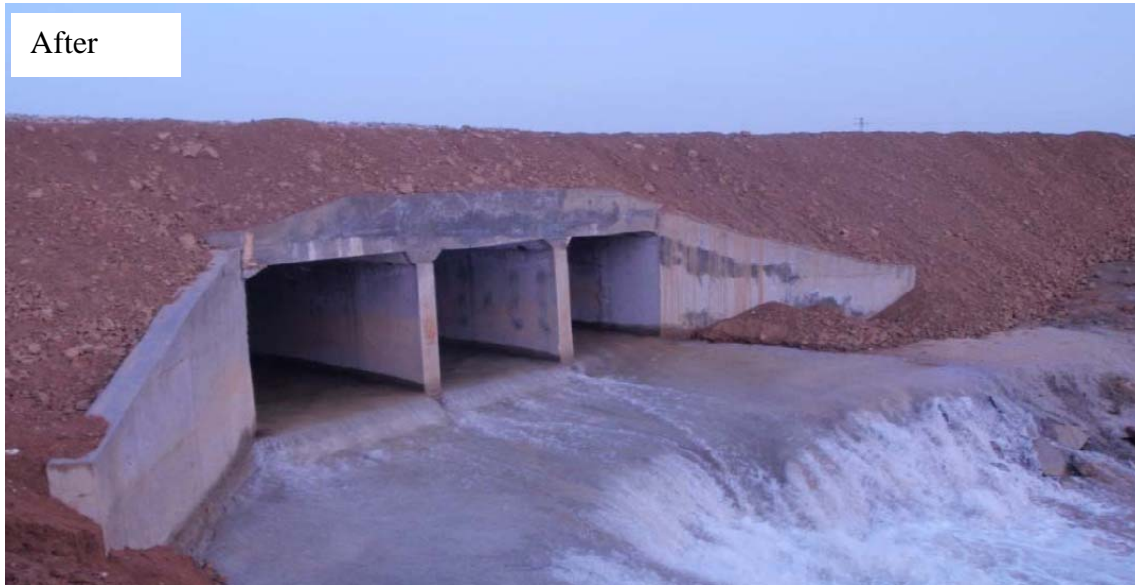
Figure 3—Qassabat Bashaar Water Culvert
