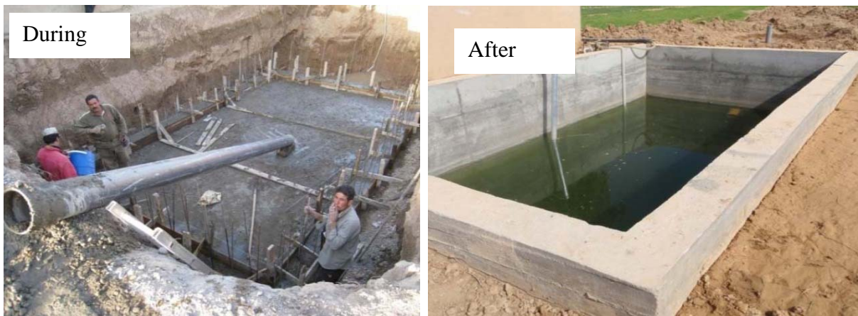
Figure 4—Al Fadoos Water Treatment Plant
