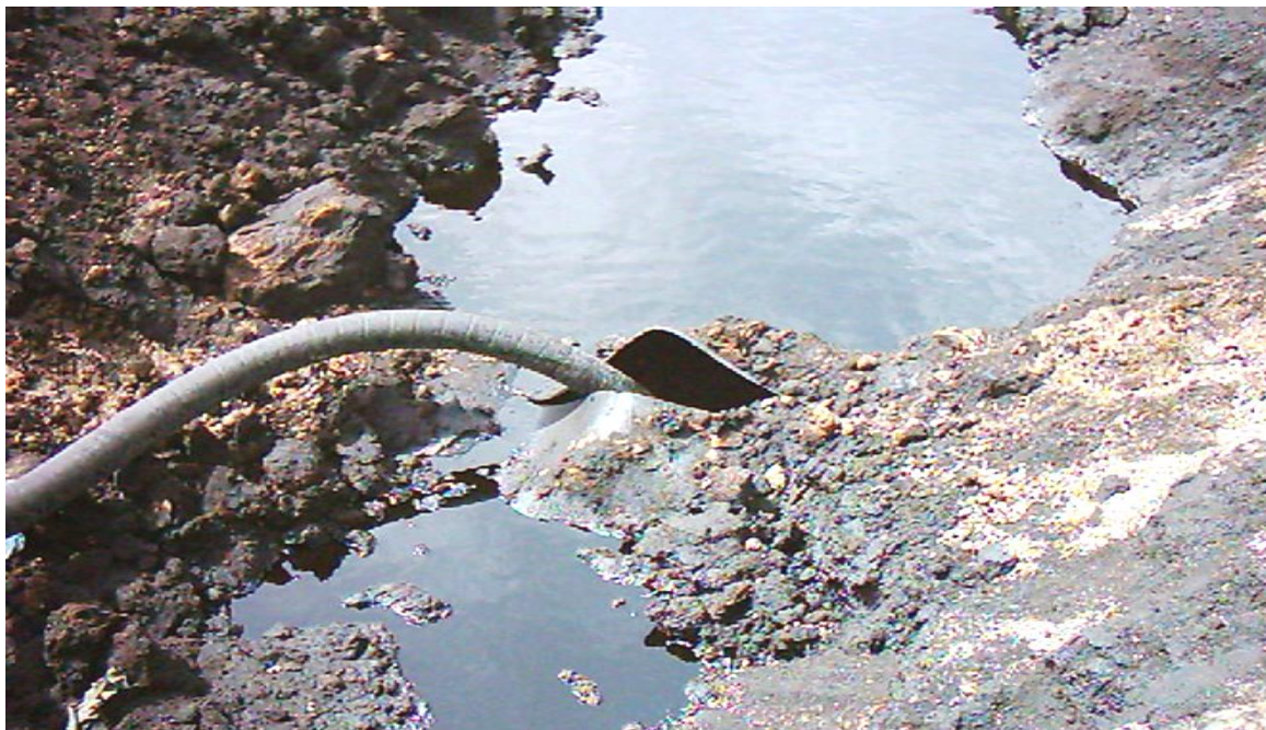
Figure 14—Task Order 19 – KBR Attempting to Pump Oil from Ruptured Pipeline
