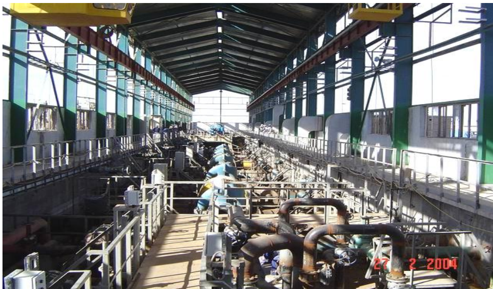
Figure 6—Ramallah Water Injection System After Repair
