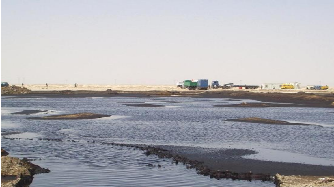
Figure 13—Task Order 19 - Ruptured Pipeline and Leakage of Oil
