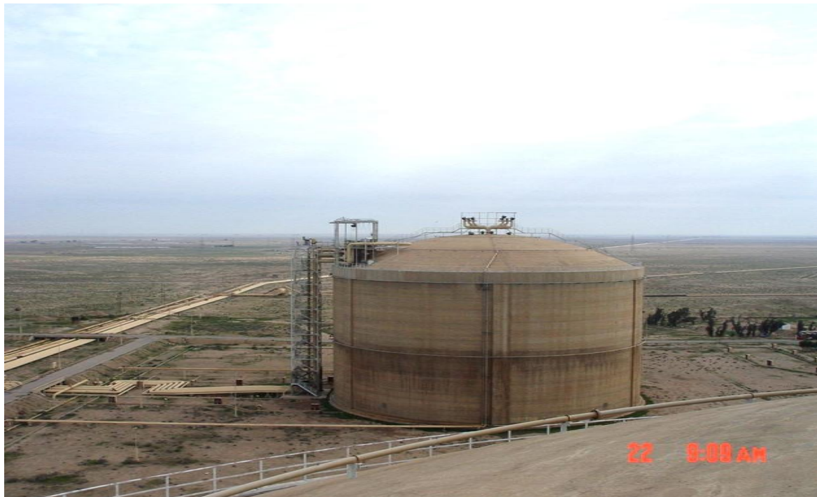
Figure 12—Cryogenic Liquefied Petroleum Gas Storage Tank at the Bulk Storage Facilities at Umm Qasr (February 2006)
