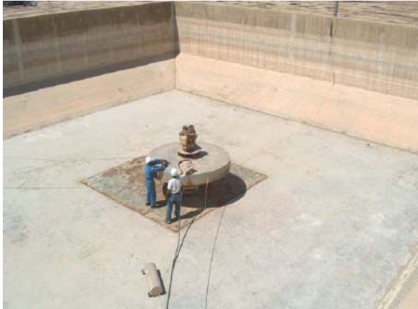
Wastewater-Treatment Plant Aerator Rehabilitation Underway
