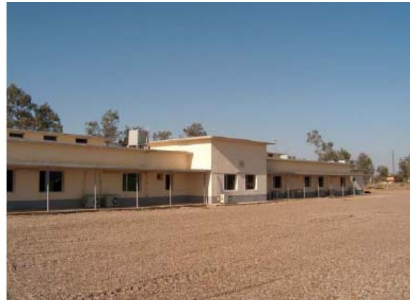
Office Building in Battalion Area After Reconstruction
