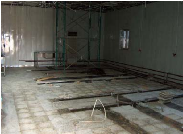
Garrison Headquarters Kitchen Before Reconstruction
