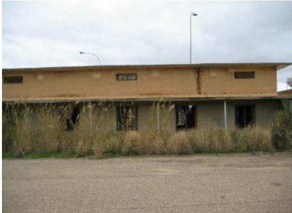
Barracks Before Reconstruction
