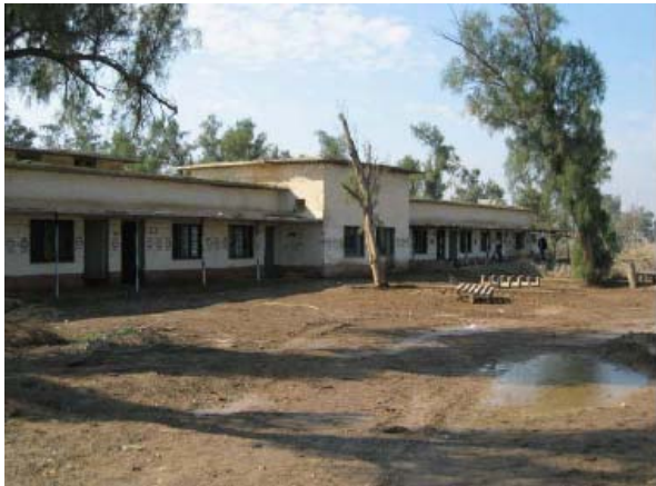
Office Building in Battalion Area Before Reconstruction
