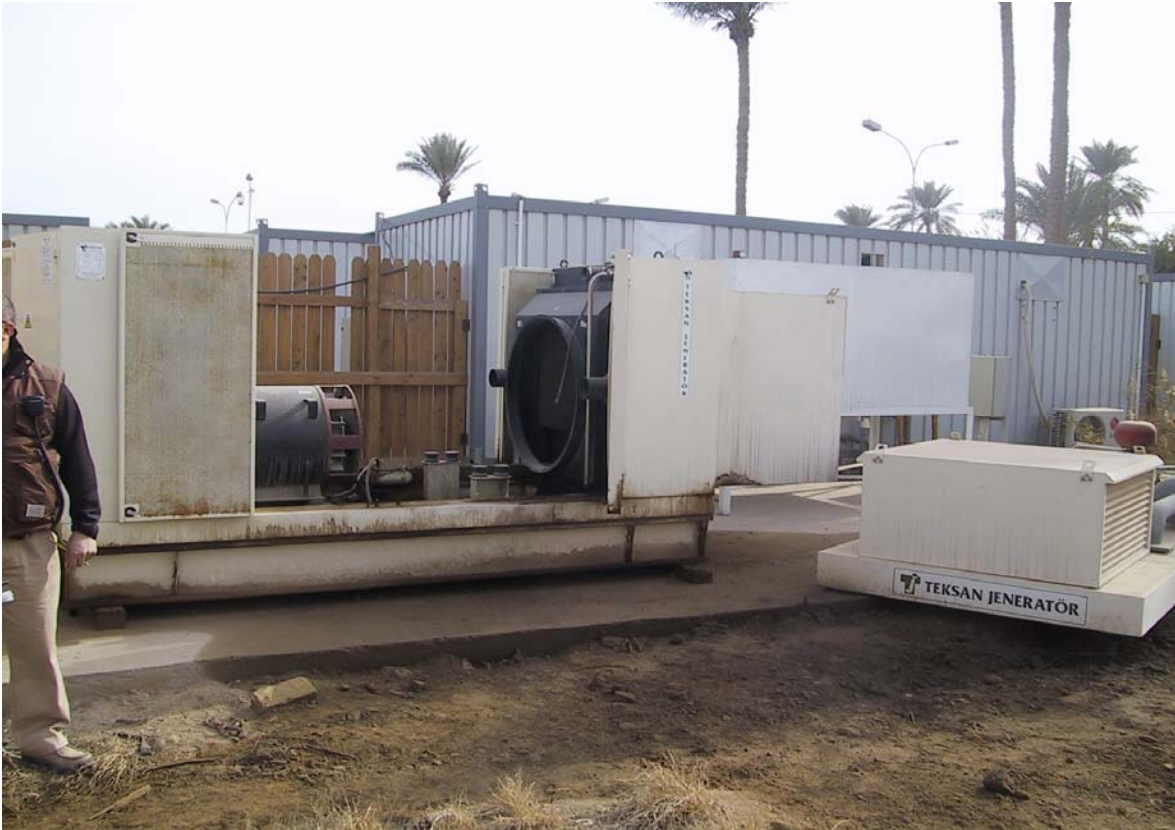
Photo 1. Shell for the 500-Kilowatt Generator Undergoing Repairs
