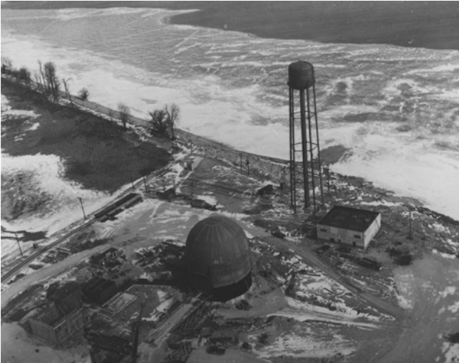
PRDC reactor under construction, 1958.
