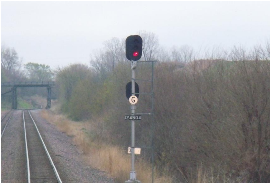
Figure 13. Eastbound intermediate grade signal 24504 with G Plate.
