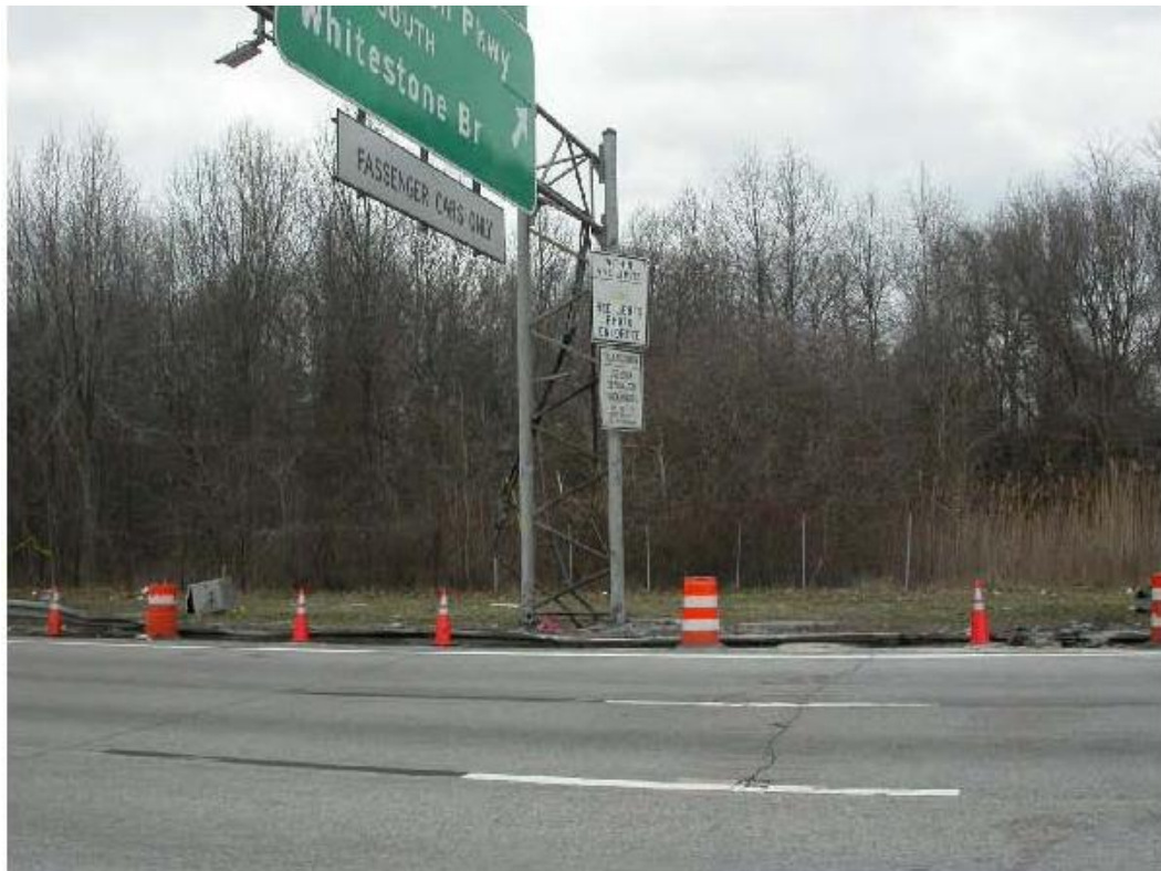
Figure 13. Overhead vertical highway signpost (east and west poles).
