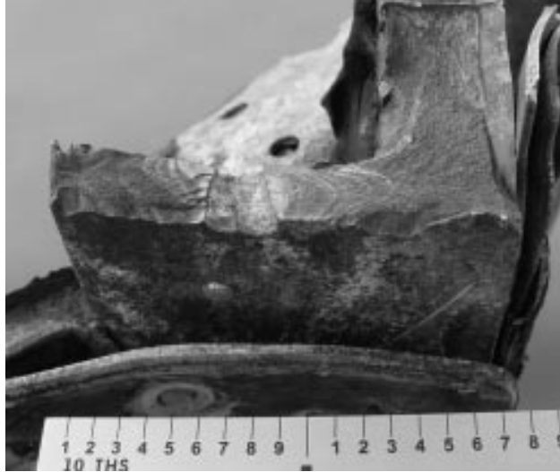
“Right-wing rear-spar lower cap fracture with fatigue cracking that initiated from a double-drilled rivet hole.”
