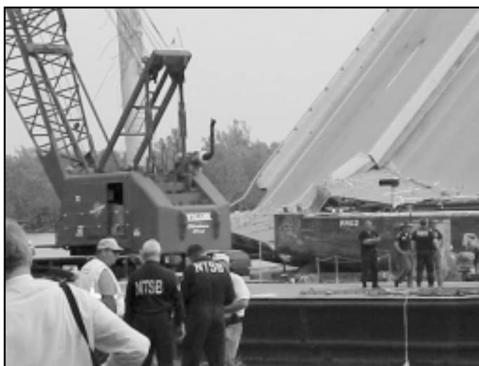
NTSB investigators on scene at Oklahoma bridge collapse.
