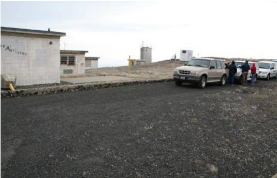
Figure A.5. 6652-C Building and Small Out-Buildings (Locale 3). Photo taken at 80 degrees on 3/19/09 by Doug McFarland.
