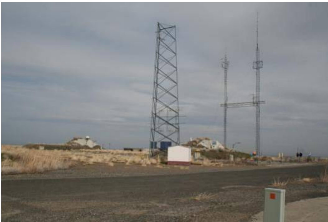
Figure A.34. Nike Bunkers and Radio Towers (Base Area). Photo taken at 20 degrees on 3/19/09 by Doug McFarland.
