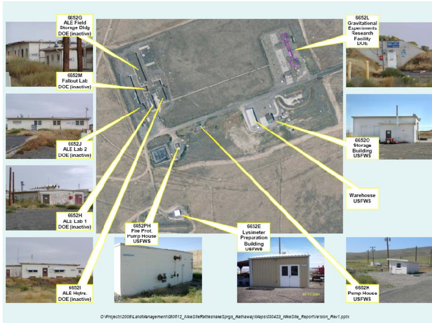
Figure 2.8. Current Facilities Located at the Former Nike Missile Base. Note the USFWS buildings that will not be demolished.
