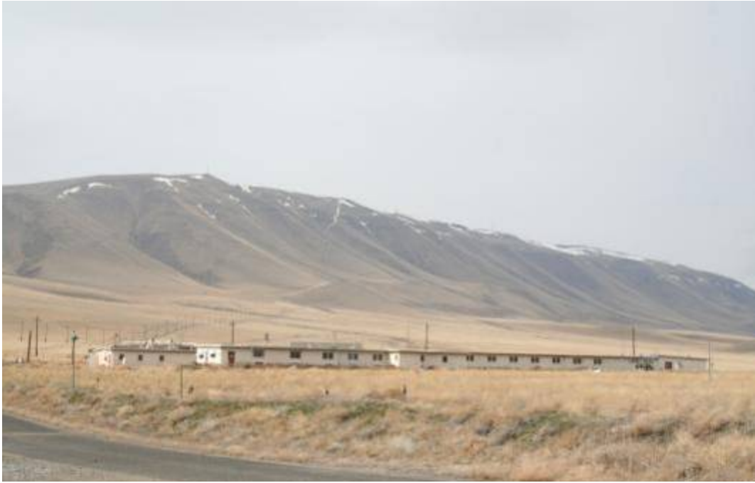
Figure A.35. Nike Buildings to Be Demolished. Photo taken at 280 degrees on 3/19/09 by Doug McFarland.
