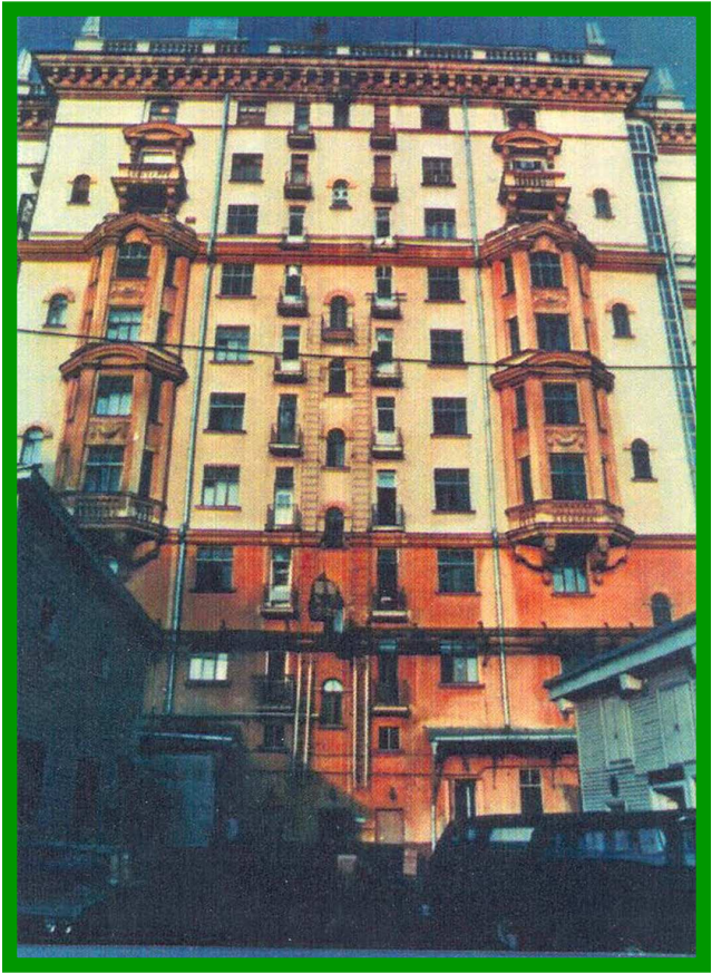
Fig. 1. U.S. embassy in Moscow. Equipment was lifted in and out of this building, possibly from the roof, since the Soviets had shut down the elevator.
