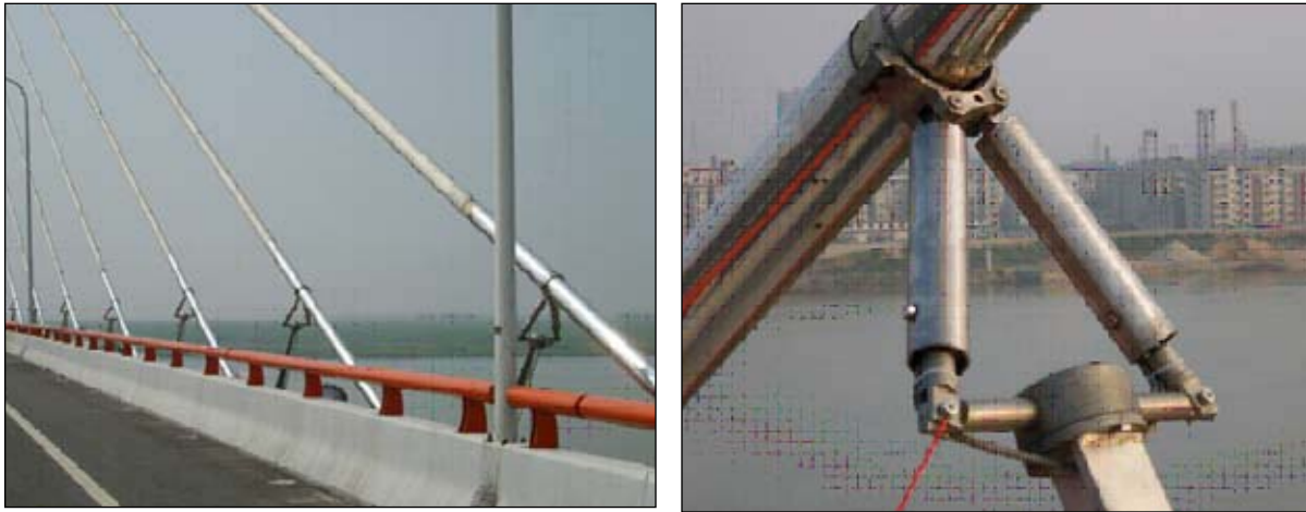
Magnetorheological dampers initially developed for the control of earthquake vibration applied to control wind- and rain-induced vibration of the Dongting Lake Bridge, Hunan, China (Spencer and Nagarajaiah, 2003).
