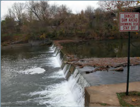
Riverton Dam before the removal
