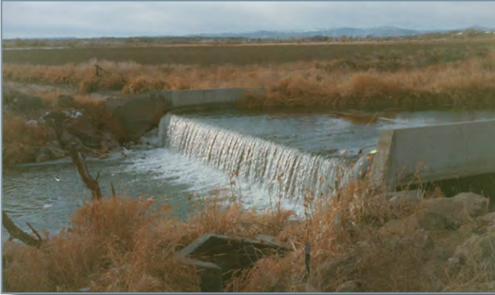
Above: The box culvert on Bitter Creek preventing fish passage.
