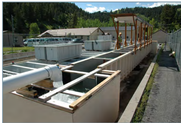
Left: In 2011 the NFPP supported the construction of a flume at the Bozeman Fish Technology Center that will be used in research on species-specific swimming capabilities to improve fish passage designs.
