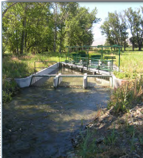
The finished diversion that prevents entrainment by fish in the irrigation canal.
