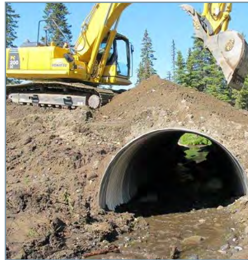
Construction of the new fish friendly culvert.
