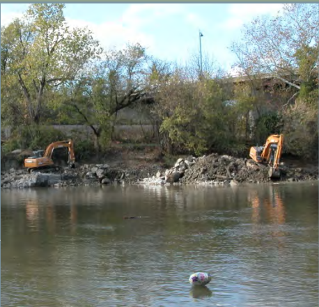
Deconstruction of Riverton Dam
