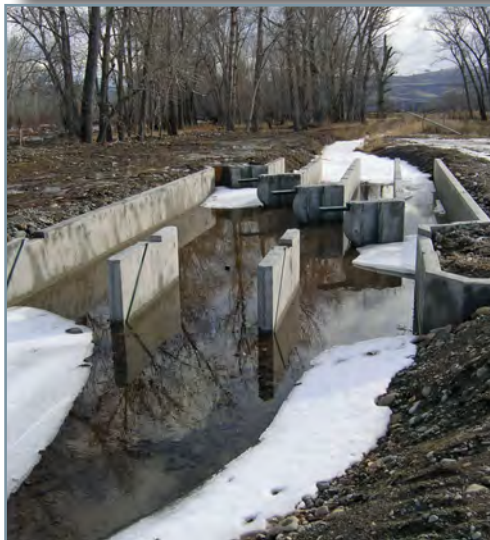
Construction of the fish screen.
