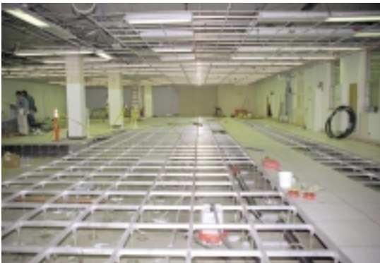
The machine room in Berkeley takes shape.
