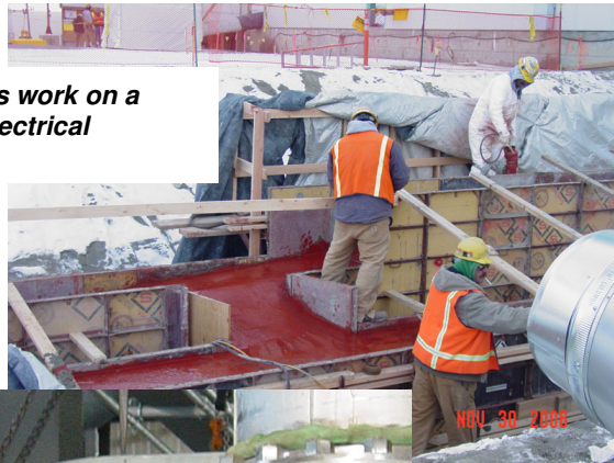
Structural steel was delivered to the Analytical Laboratory at the Construction Site in late November. Erecting structural steel is a significant milestone in the construction of the full-service laboratory.
