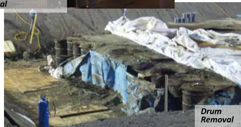
Trench 7 Drum Retrieval
