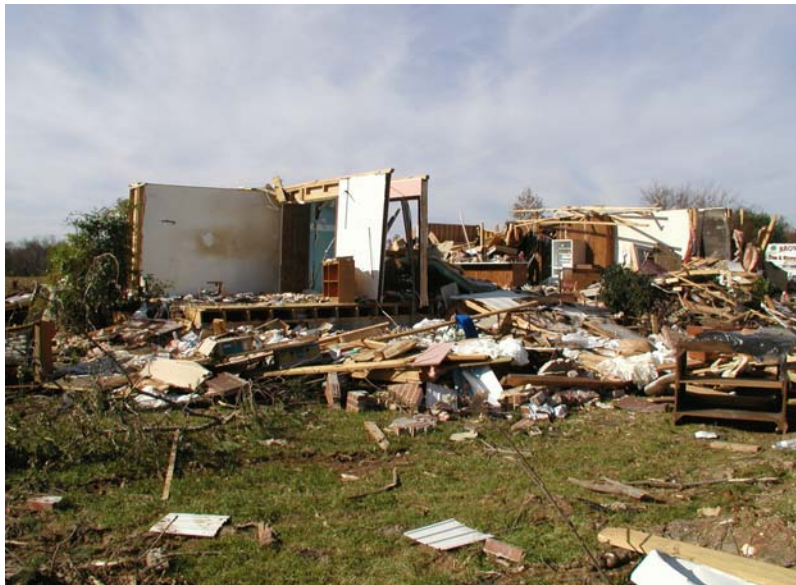
Remnants of house struck by an F3 tornado in Mossy Grove, Tennessee, on November 10, 2002. (NOAA)
