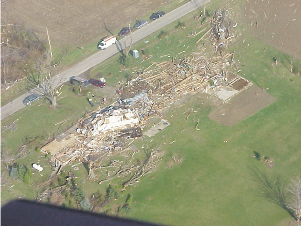
Aerial view of F3 tornado damage to homes near Republic in Seneca County, Ohio, on November 10, 2002. (NOAA)
