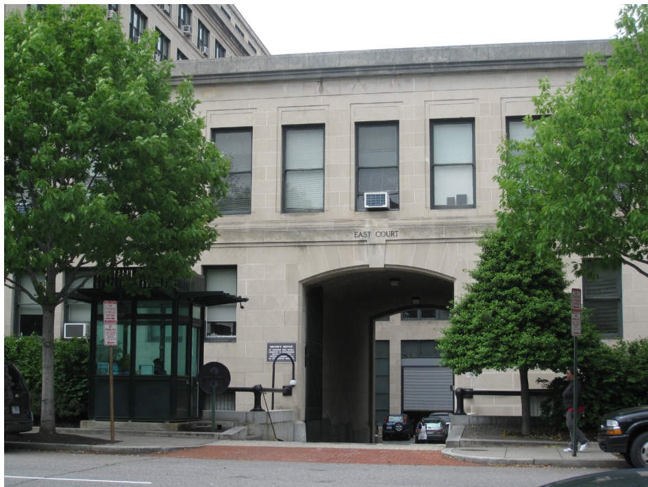
Figure 3-3d: Courtyard Entrance on South Side of 1800 F Street Federal Building
