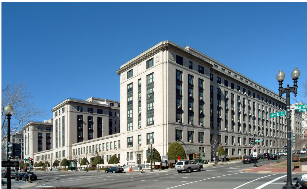
Figure 2-1: Existing 1800 F Street NW Federal Building
