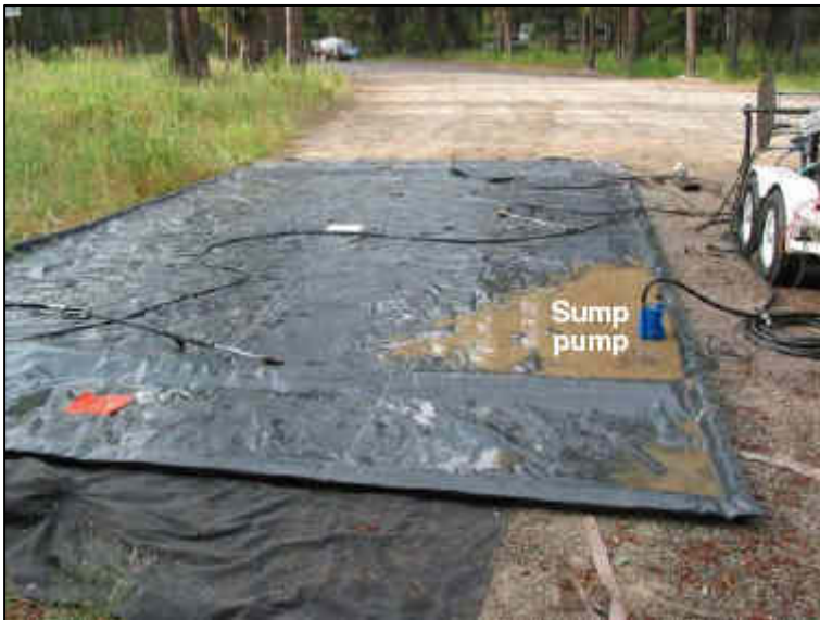
Figure B-1. Bermed portable mat system with sump pump for water recycling (U.S. Department of Agriculture, Forest Service site).
