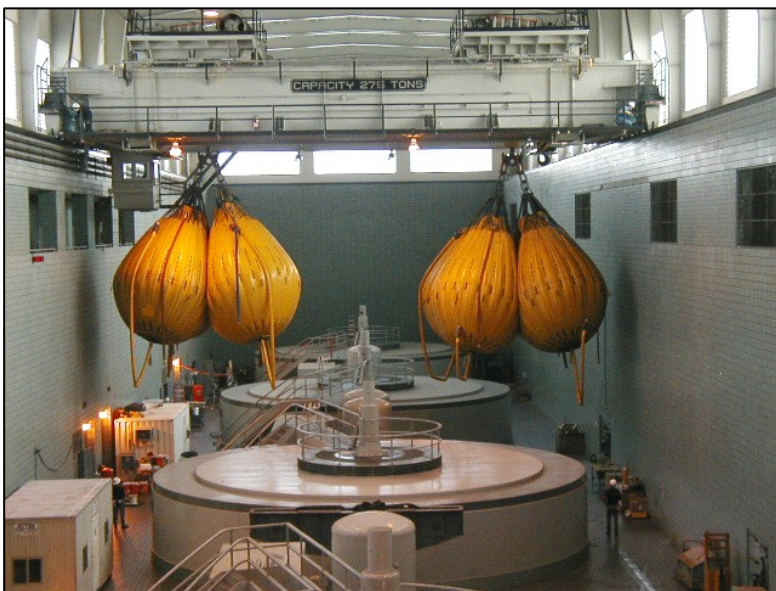
Figure 12. Crane being tested at a Tennessee Valley Authority powerplant using water weight bags™ (photo by Mike Hoffman; photo courtesy of Jim Jota, Imes, Inc., 2002).
