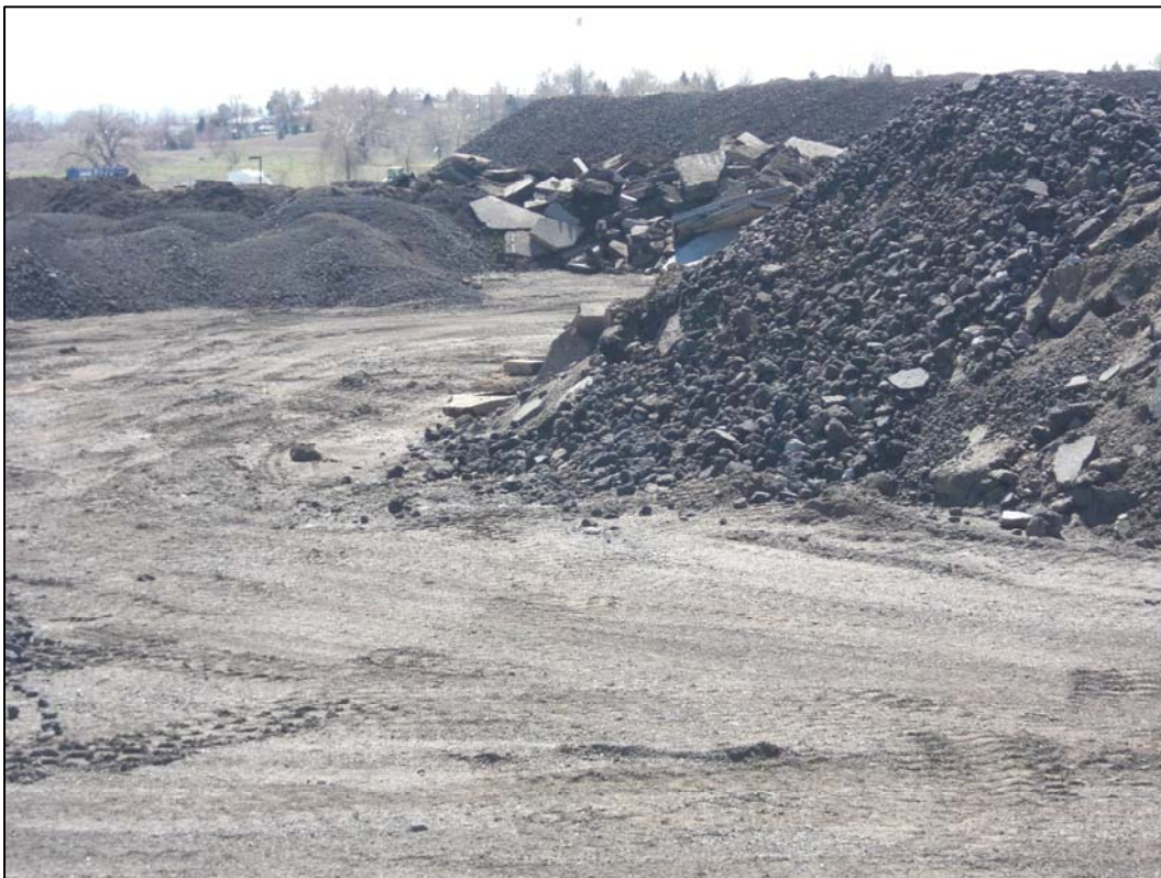
Figure A-1. Fill materials separated by type – soil, broken concrete, pavements, etc. – temporarily stored at a barrow site (photo courtesy of Joe Divittorio, 2010).
