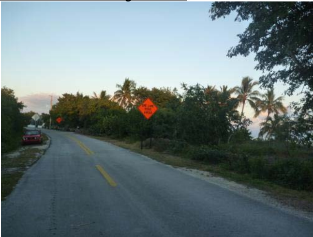
Boca Chica Beach roadway between beach and NAS Key West - 6 months after treatment
