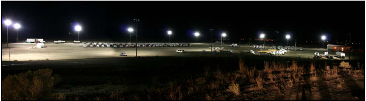
This photo taken in the early morning shows the lighted transportation yard at the Environmental Restoration Disposal Facility. The transportation yard is used by the truck and pups. (Photo 3)
