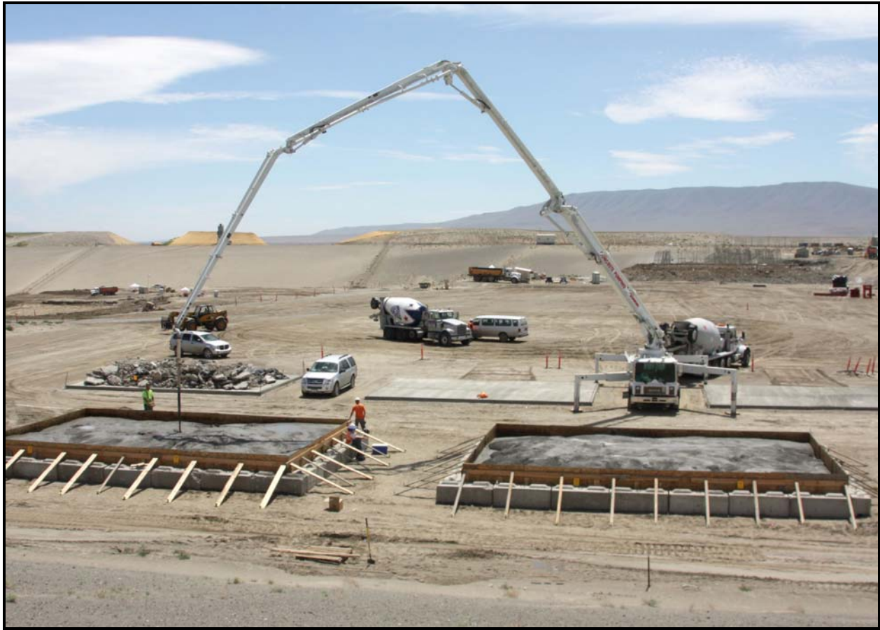
The Waste Operations team at ERDF constructed macro pads to dispose of chromium-contaminated debris. (Photo 5)
