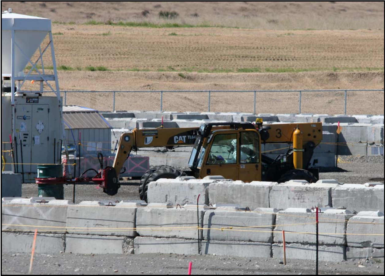
A telehandler moves a concreted drum at the 618-10 Burial Ground. (Photo 9)
