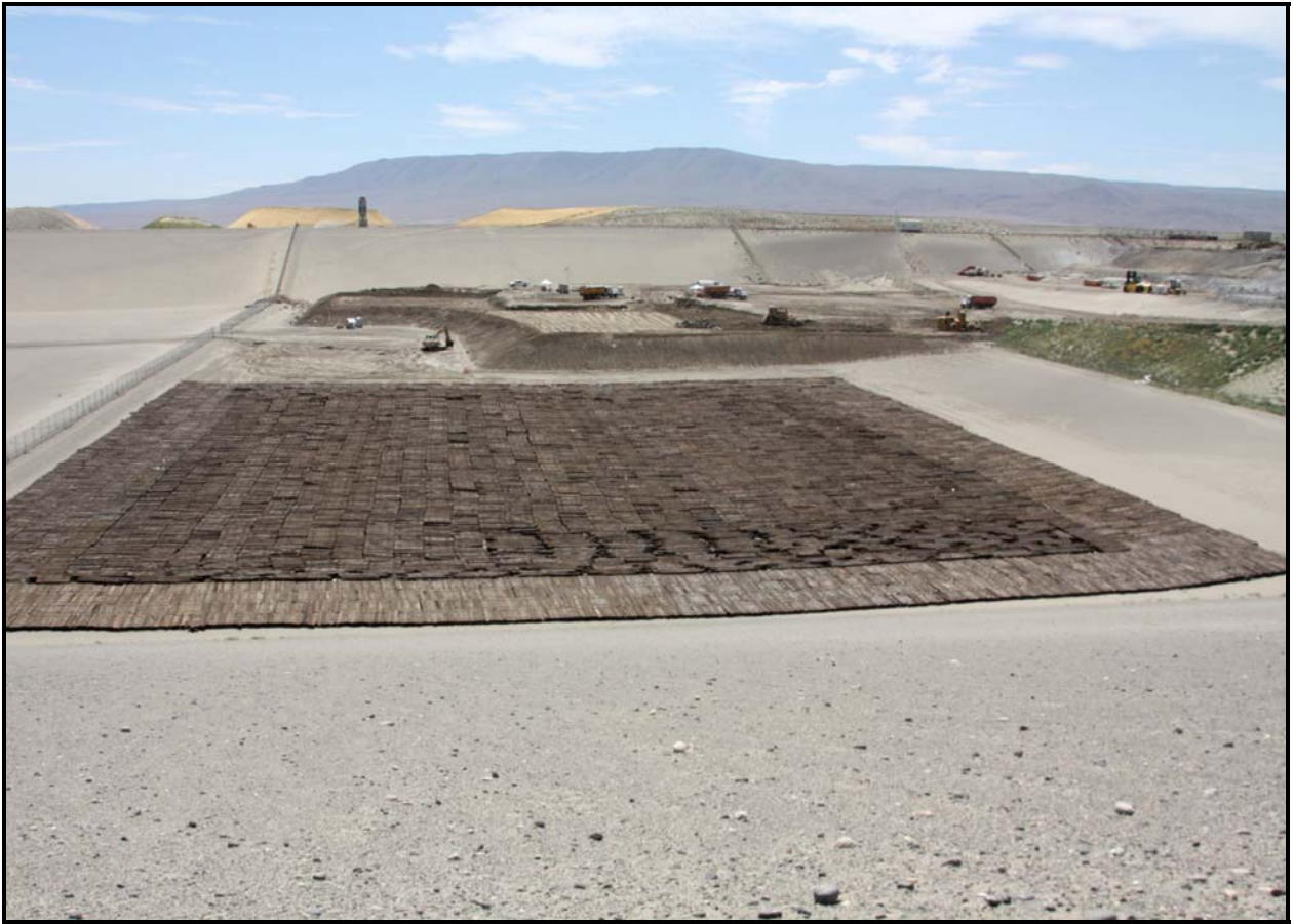
Earlier this month, ERDF received the final shipment of 58,500 Hanford Site railroad ties for disposal. (Photo 4)
